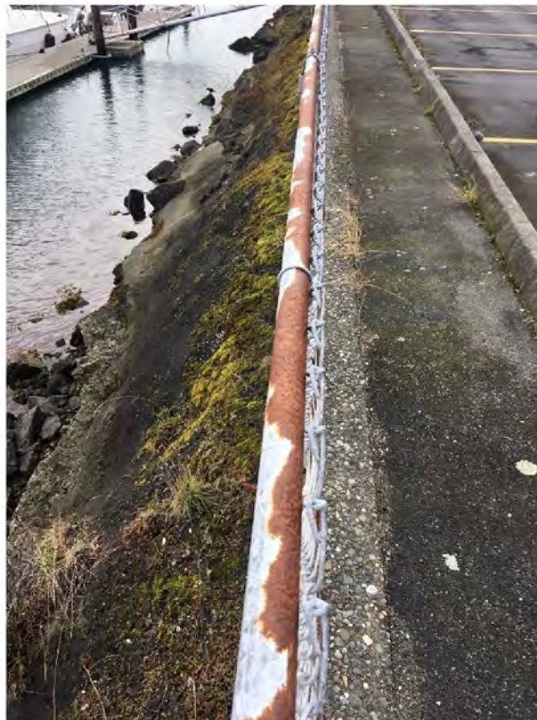
Existing concrete bulkhead, shotcrete, and rip rap below. Paved & fenced parking lot above.
