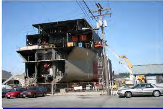
Ship Building at Marine Terminal
