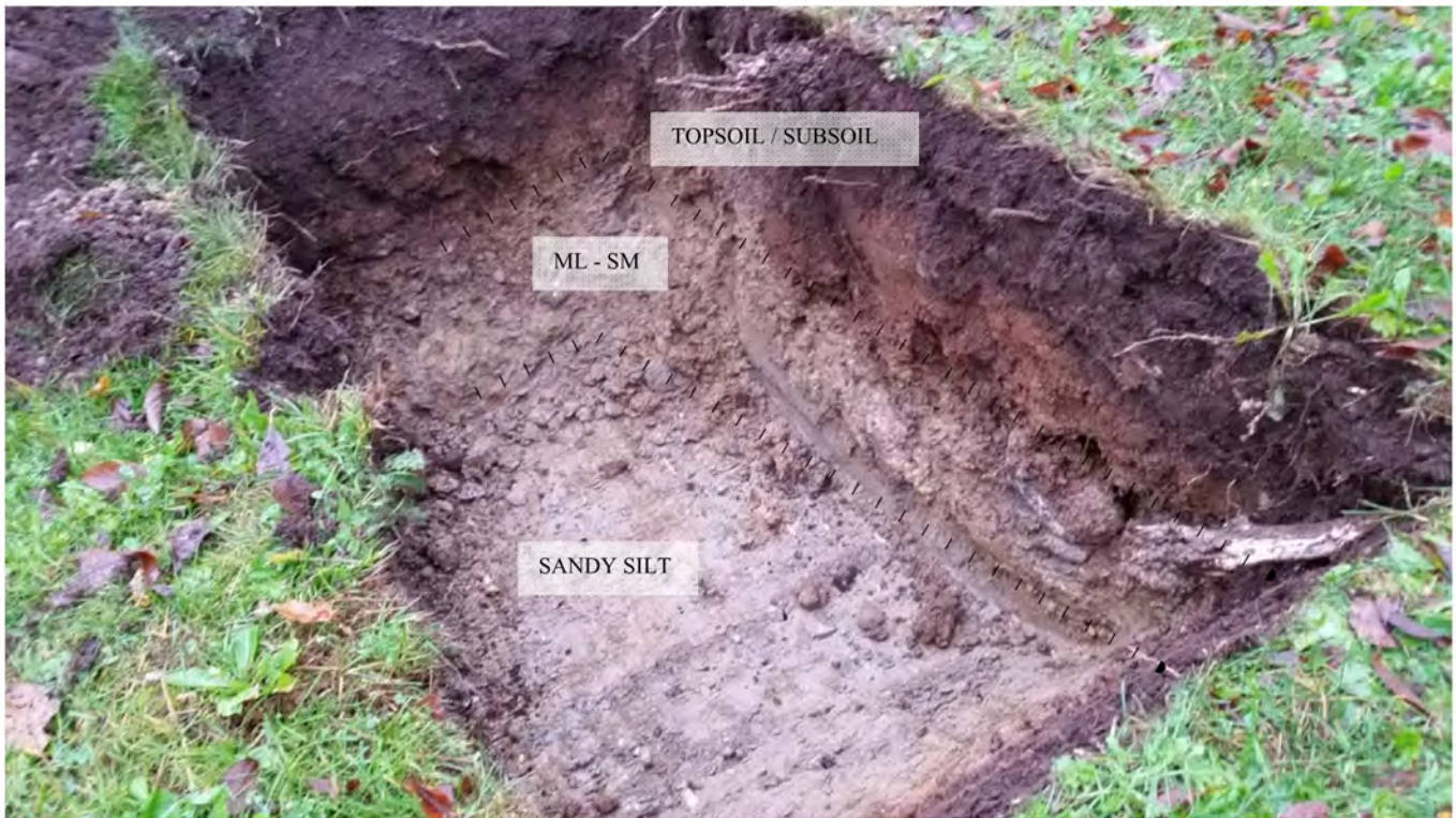
Photo C: Representative soil stratigraphy as viewed at TP-3 location in progress.
