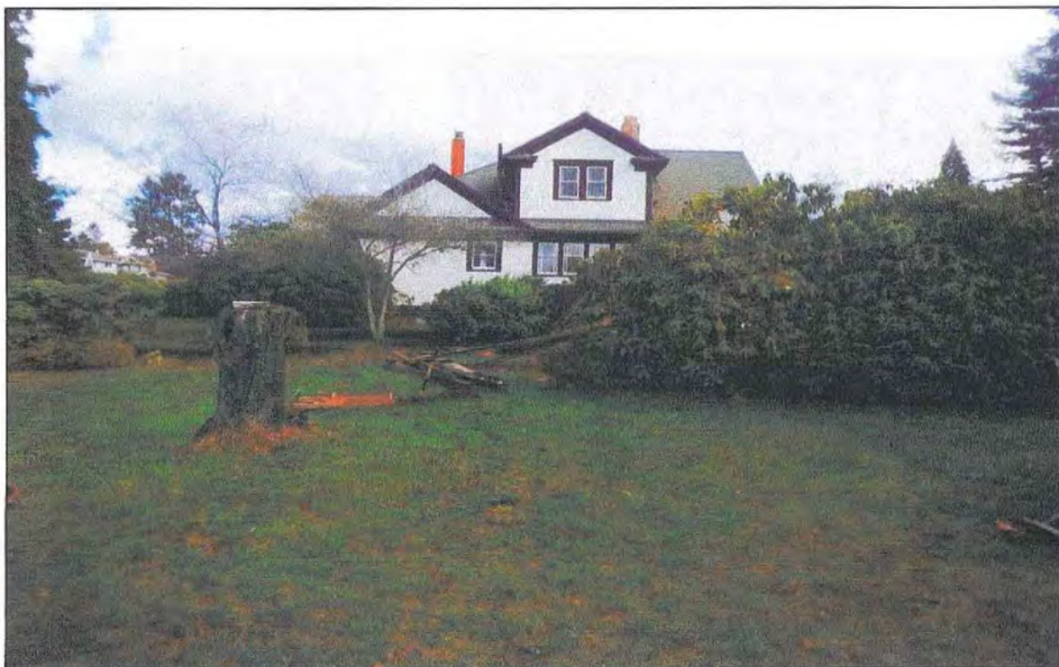
Photo 1. Overview, rear and south, of the residence from the orchard area.
