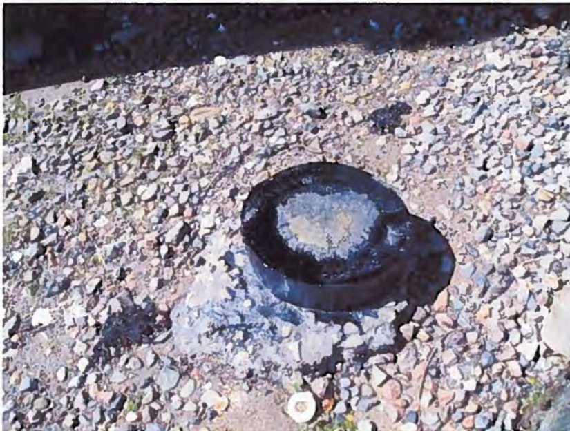
Another piling, cut, but still leaching creosote.
