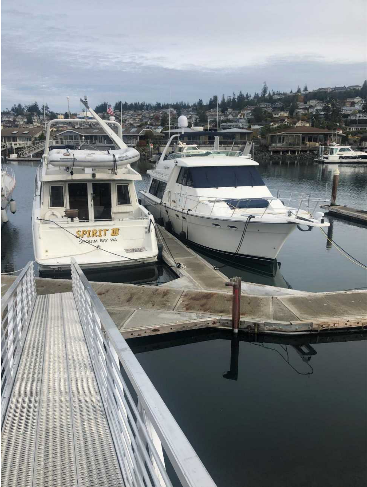
Existing Stand-Pipe Fire Extinguisher Connection Example-No Change
