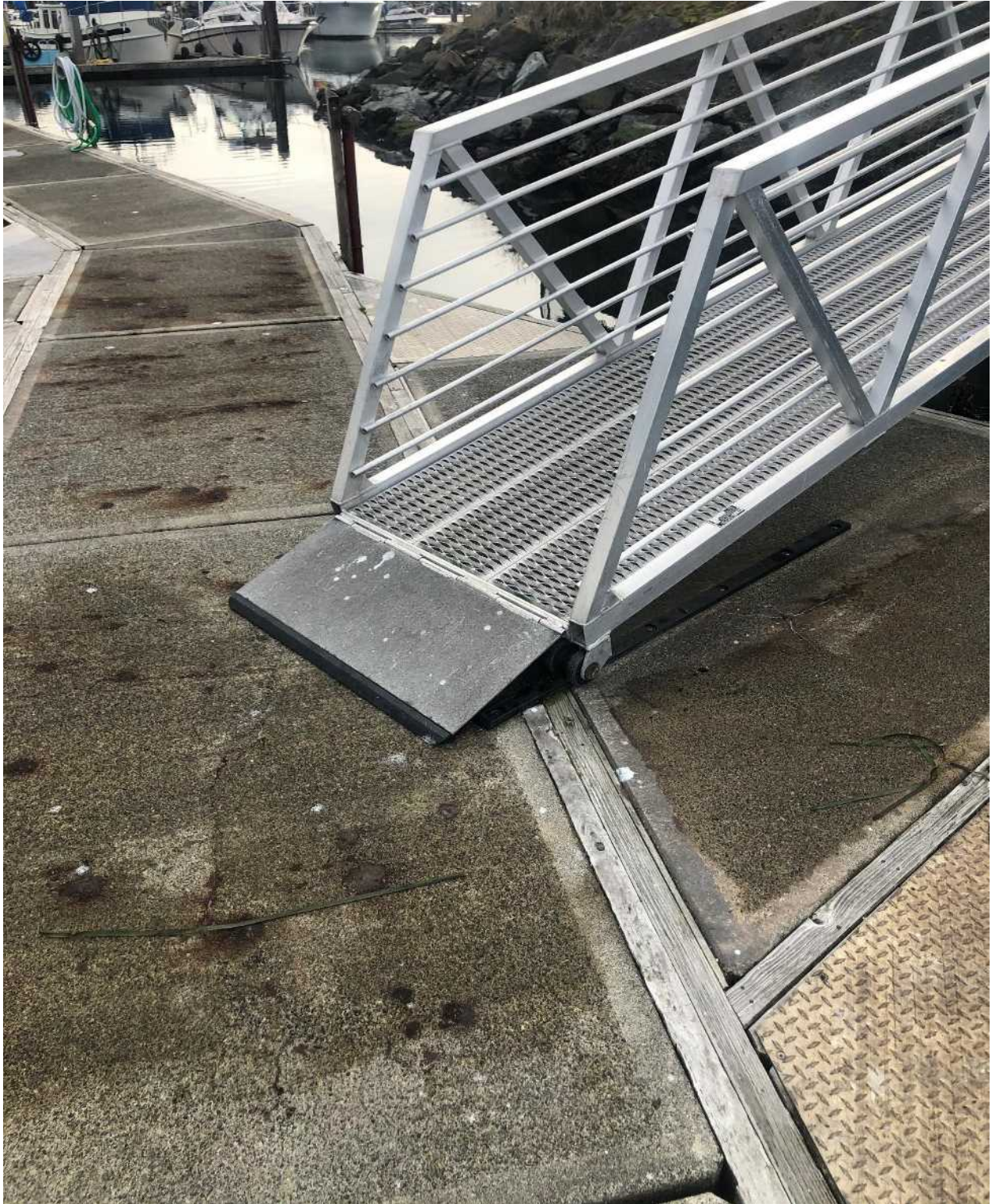
Example-Ramp from Land Connects to Float(s) on Rollers-Unchanged
