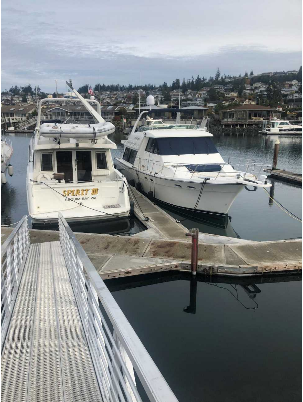
Existing Stand-Pipe Fire Extinguisher Connection Example-No Change
