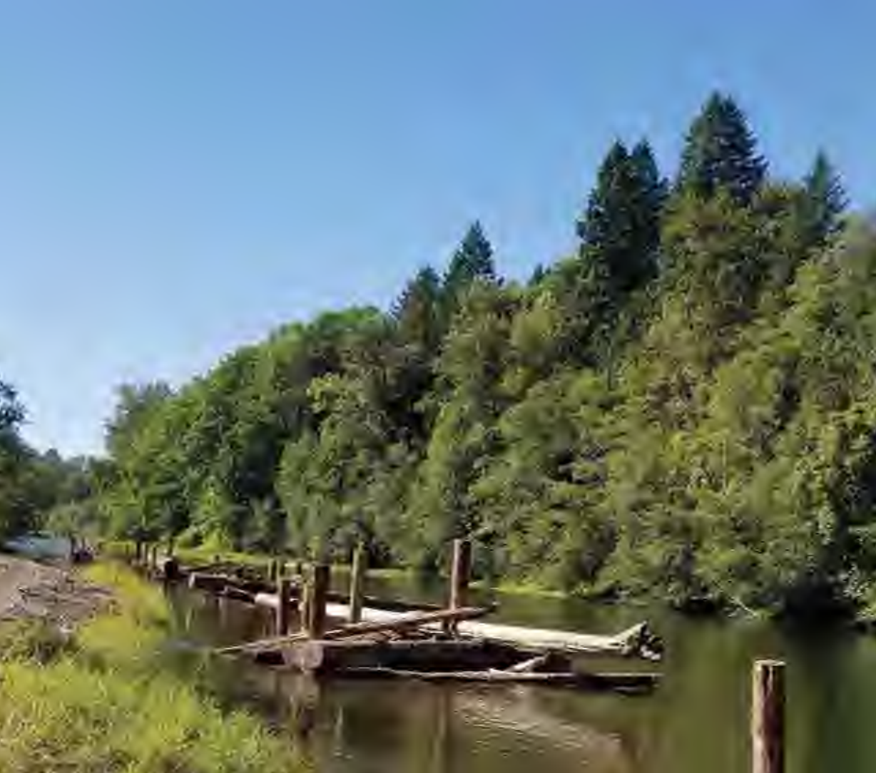
Engineered large wood structure in the north fork of the Lewis River/ Chuck Stambaugh, WDFW
