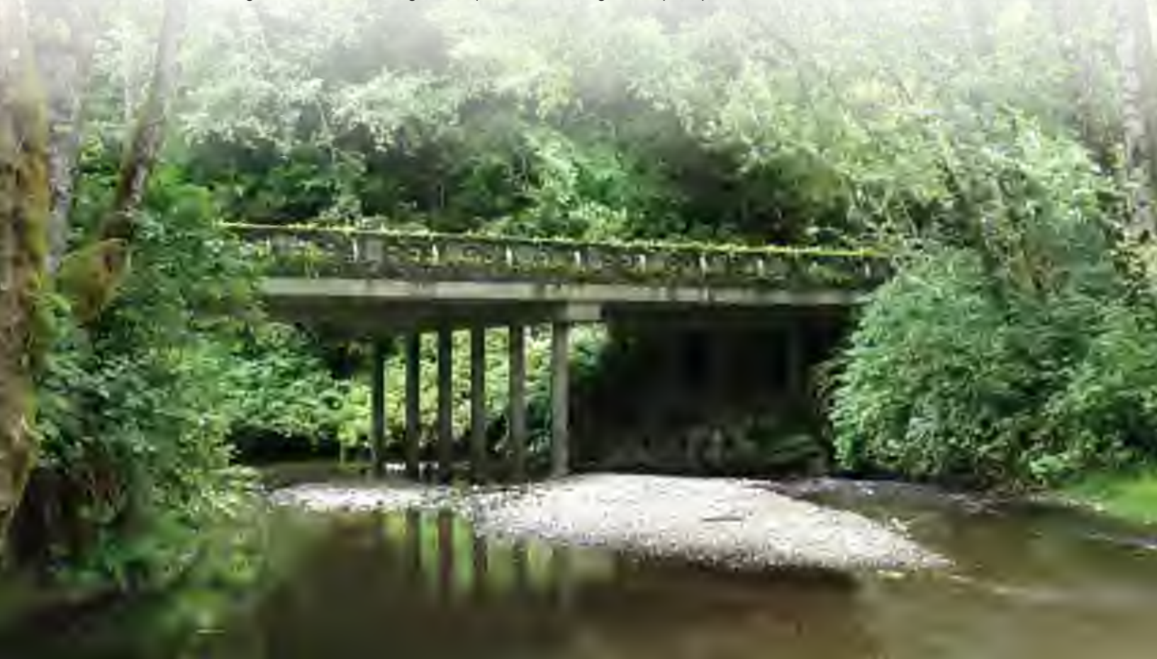
Bridge on Strait of Juan de Fuca Highway/Ned Pittman, WDFW
