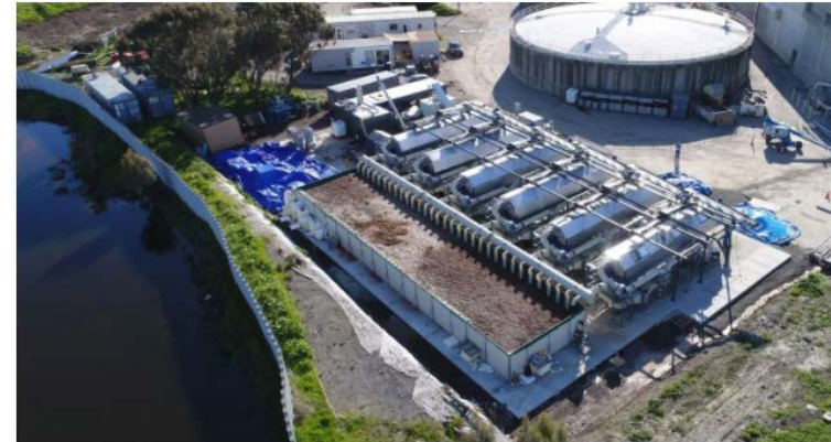
Aerial view of BioForceTech's plant in Silicon Valley, California, US
