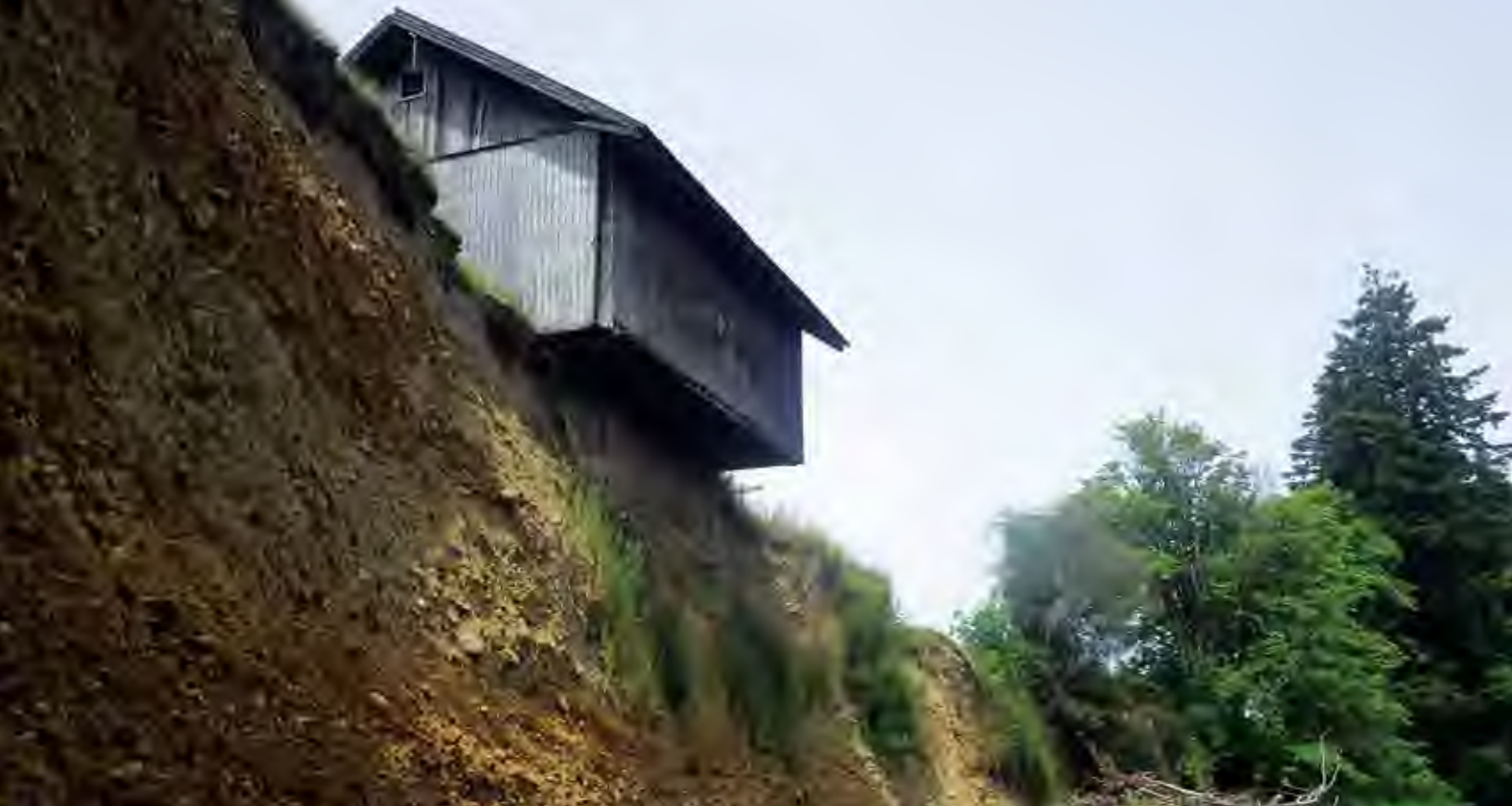
Building in danger from streambank erosion on Newaukum River/Kaysie Cox, WDFW
