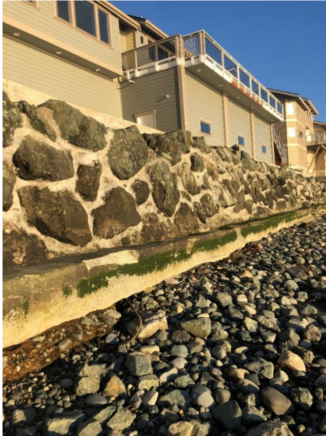
Figure 2. Photo of existing bulkhead and exposed toe
