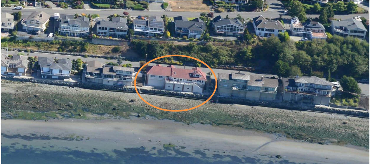
Figure 15. WECY Shoreline Aerial Photo (8/18/2016)
