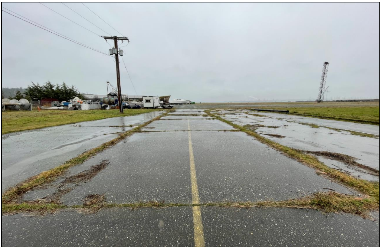
Photo 2. Eastern overview of the proposed road at the connection to 17th Street.
