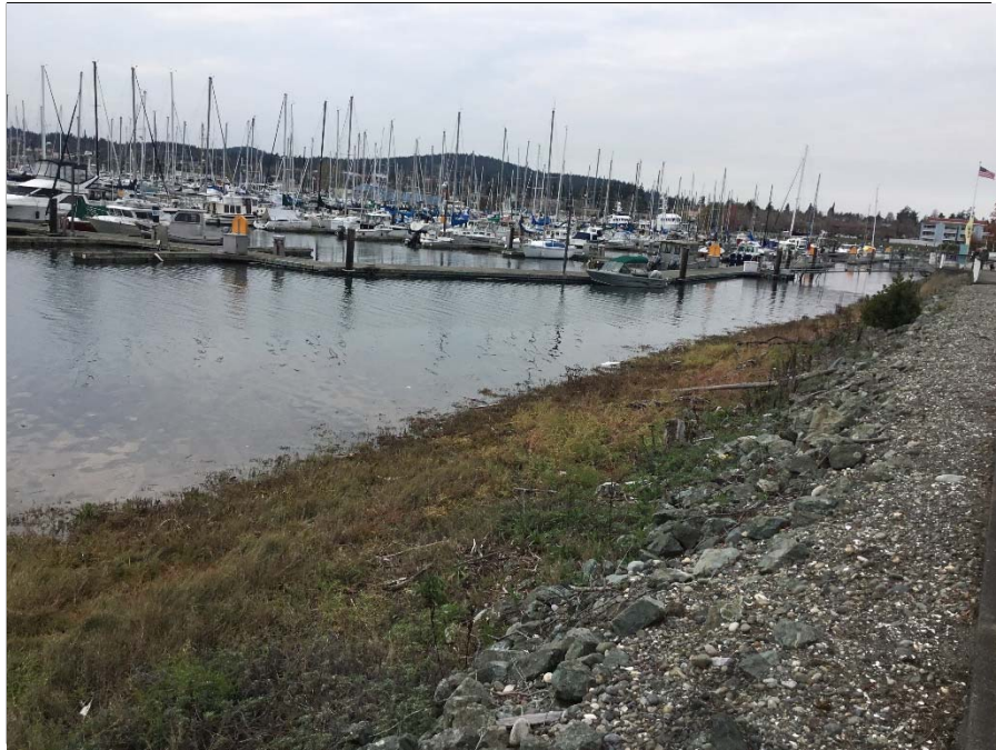
Photograph 5. Looking west along the armored shoreline.
