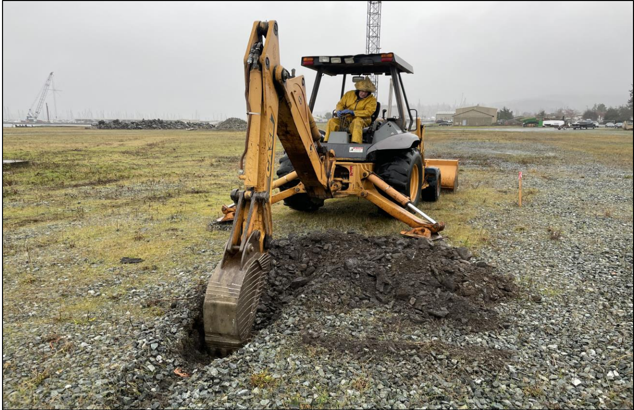
Photo 7. An overview south during trenching.
