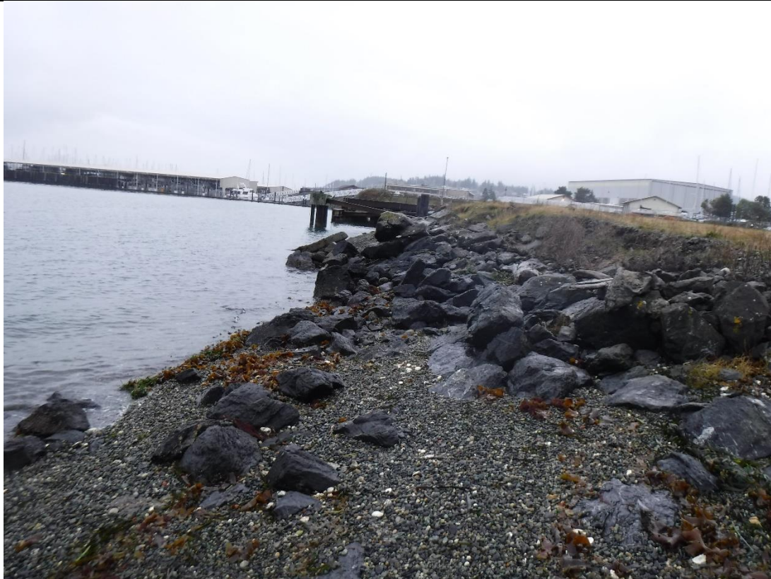
Site Shoreline, beach—mixture of boulders and pebbles—Facing South
