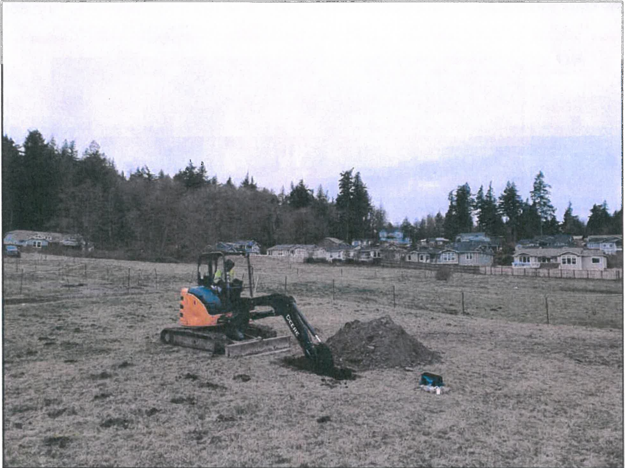
Image 1. View of the excavation process at test pit # (TP-#) showing the typical overall site conditions.
