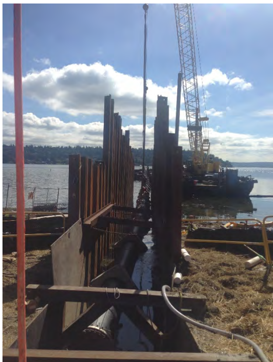
Figure 3-2. Outfall construction using sheet piles
