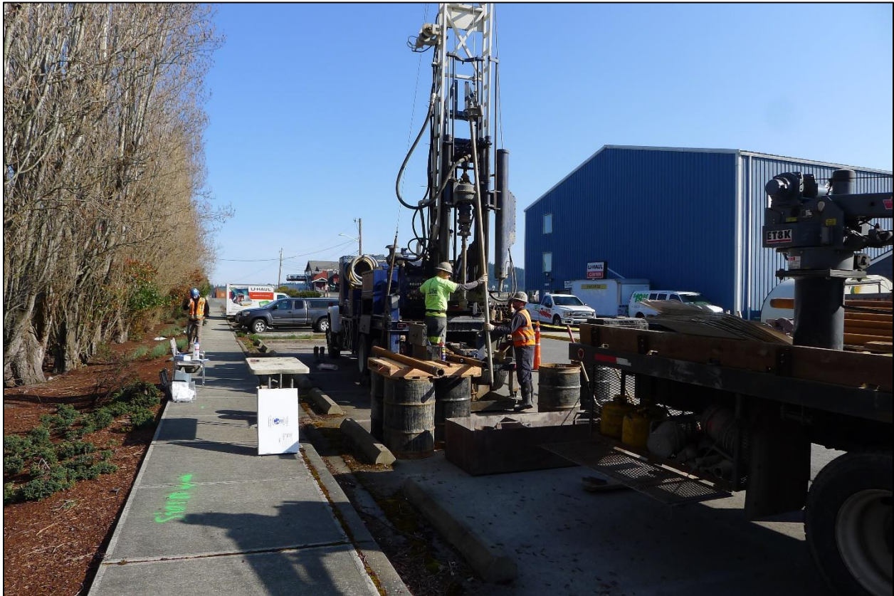
Photo 1. The first drill hole location, viewing north up T Avenue.
