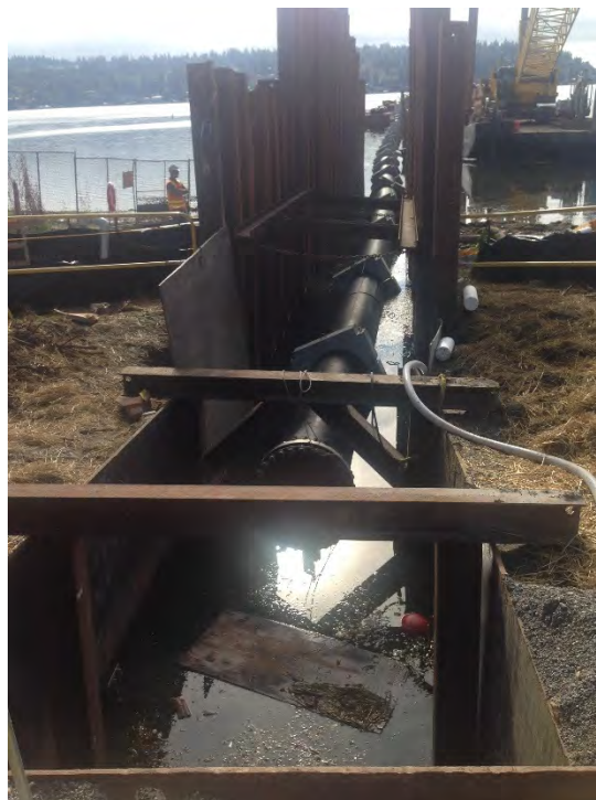
Figure 3-2. Outfall construction using sheet piles
