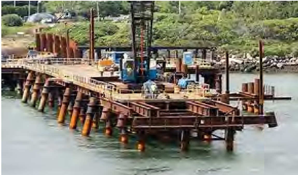
Figure 3-2. Outfall construction using sheet piles
