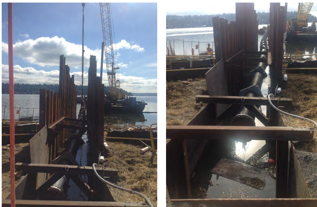
Figure 3-2. Outfall construction using sheet piles
