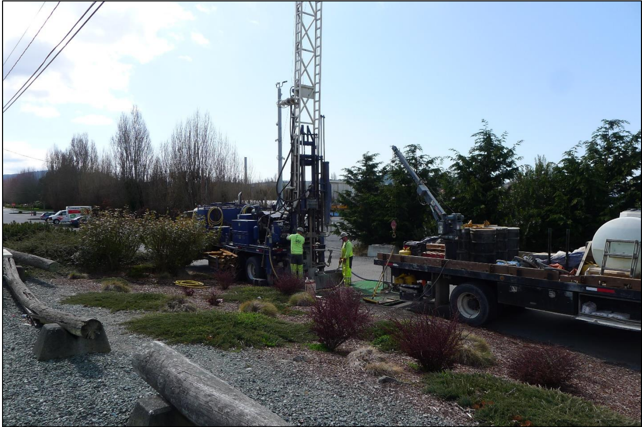
Photo 4. The second drill hole location, viewing southwest.
