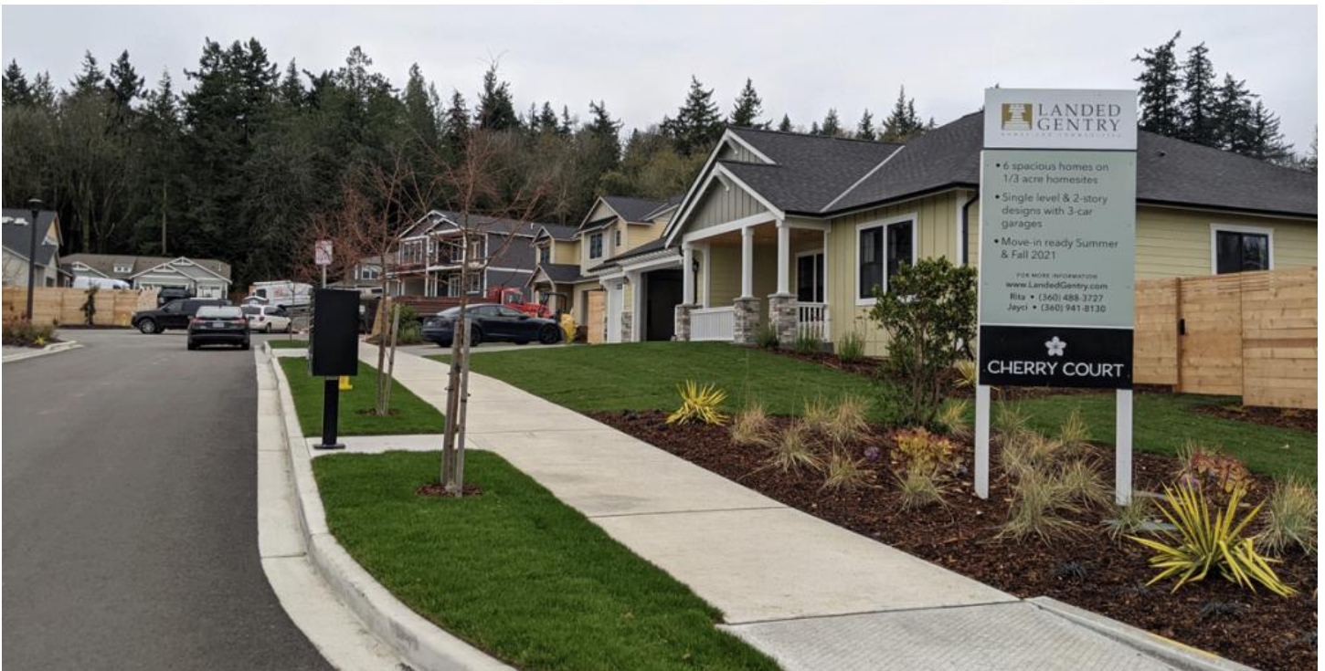
New single family homes under construction in Anacortes. Photos Eric Hall
