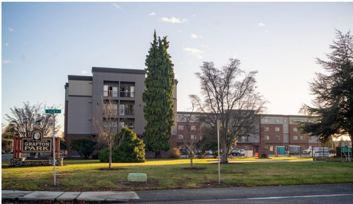
The Grafton Park Apartments are a 140-unit apartment complex with ground-floor commercial space under construction on Burlington Boulevard across from Fred Meyer. Photo Eric Hall
