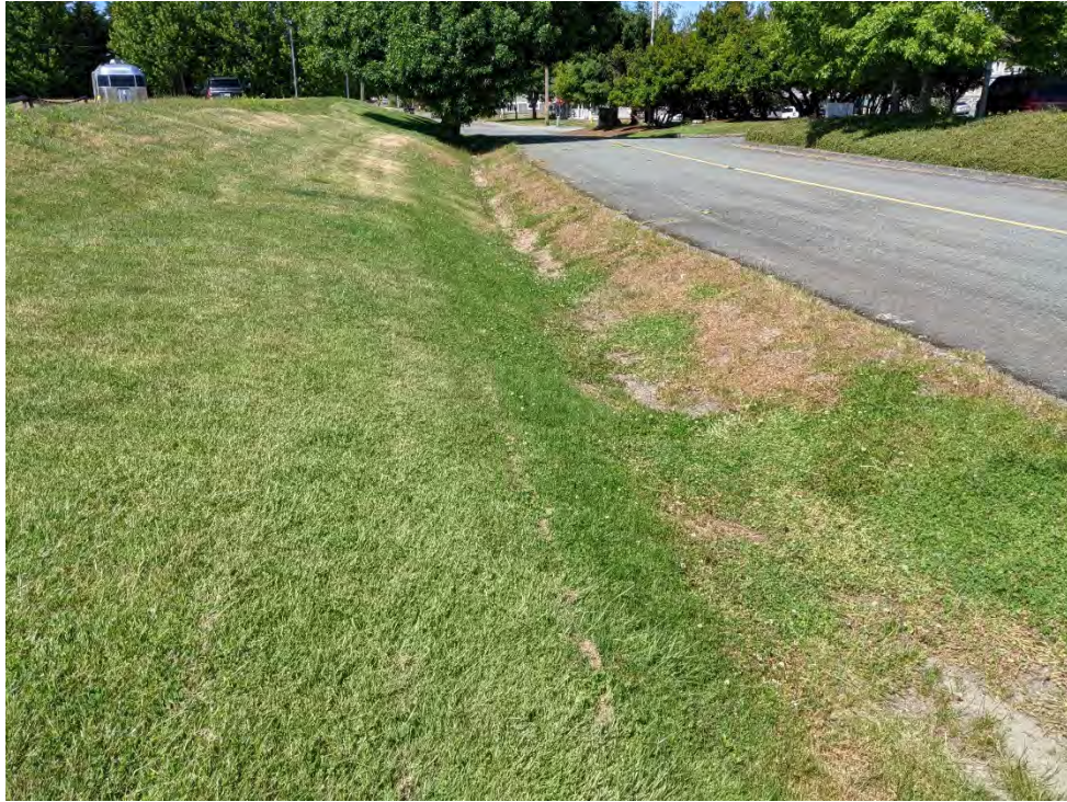
Image 3: Existing ditch on west side of T Ave, looking North
