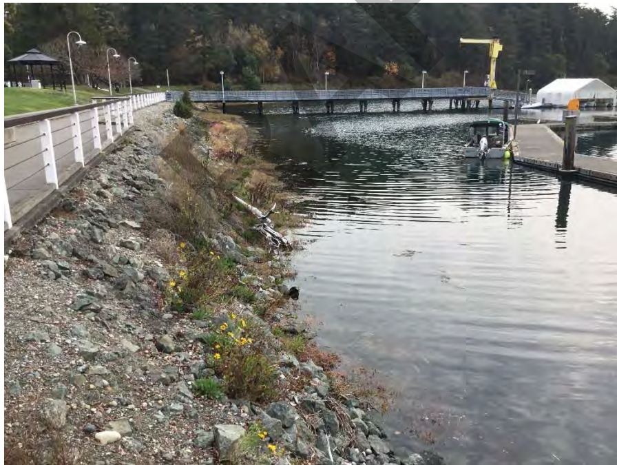
Photograph 6. Looking east along the armored shoreline; vegetated areas begin to transition to bare riprap.
