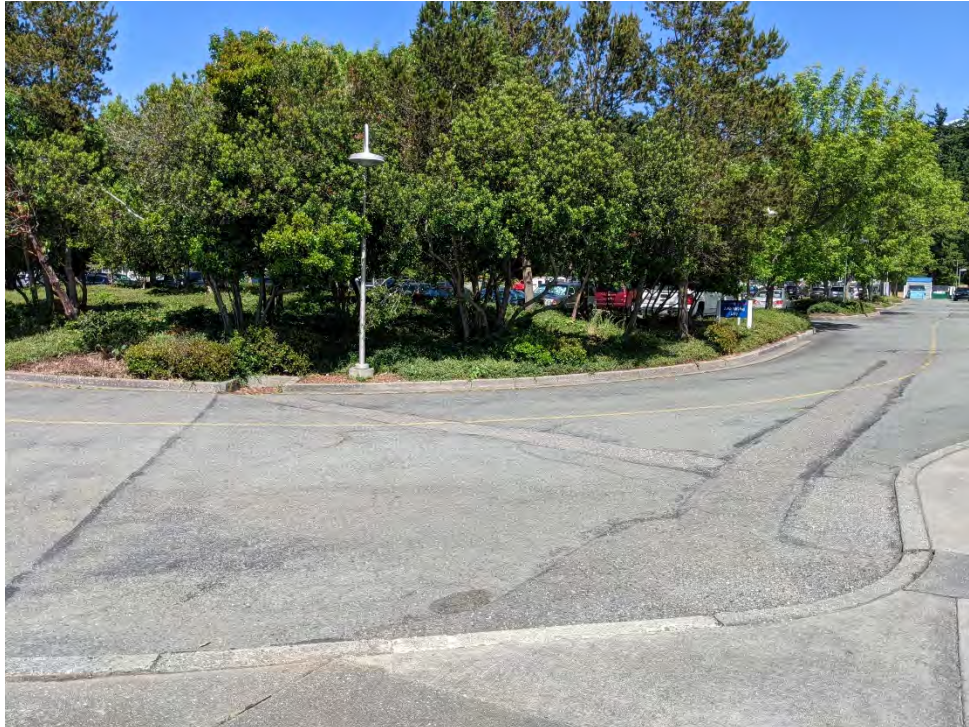
Image 1: SDCB at SE Corner of Project Site on T Ave, looking East
