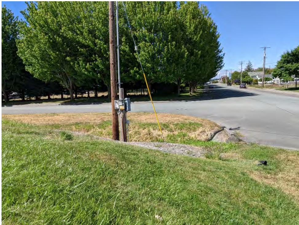
Image 4: Drainage at the SW corner of T Ave & 6 th St , looking North
