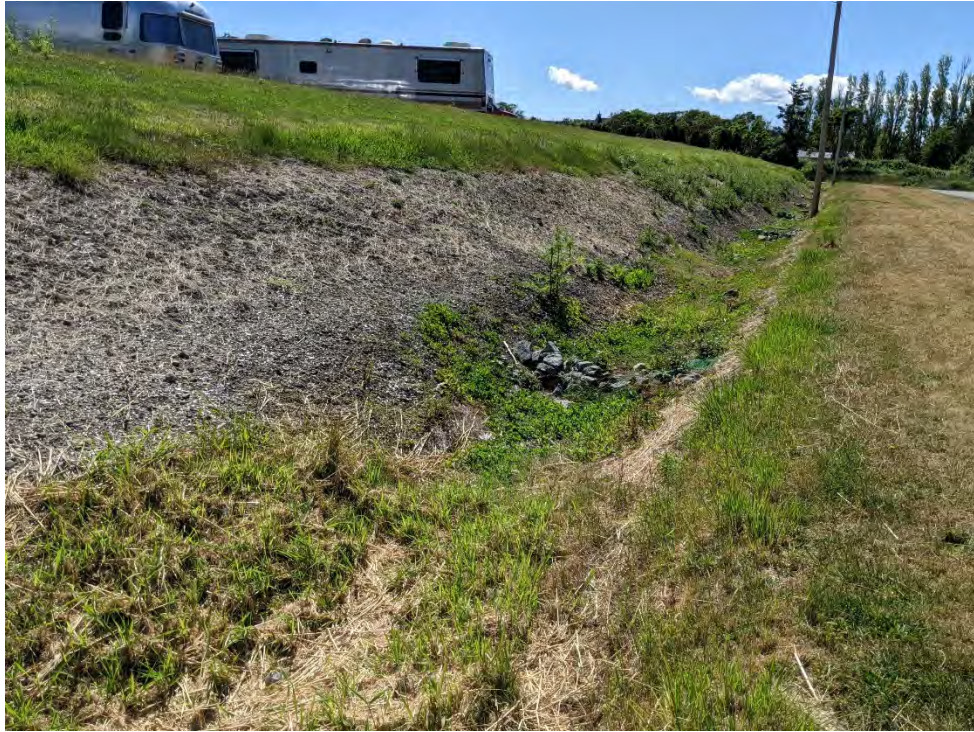
Image 7: Ditch on South side of 6 th St, looking West
