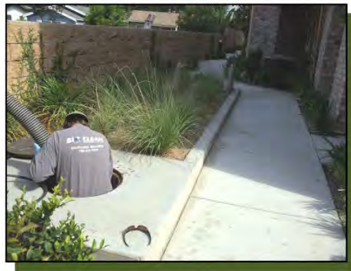
Vacuuming out of media filters.
