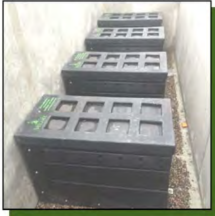
Pre-filter cartridges with tops on.
