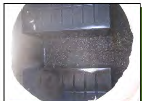
Fully cleaned separation chamber.
