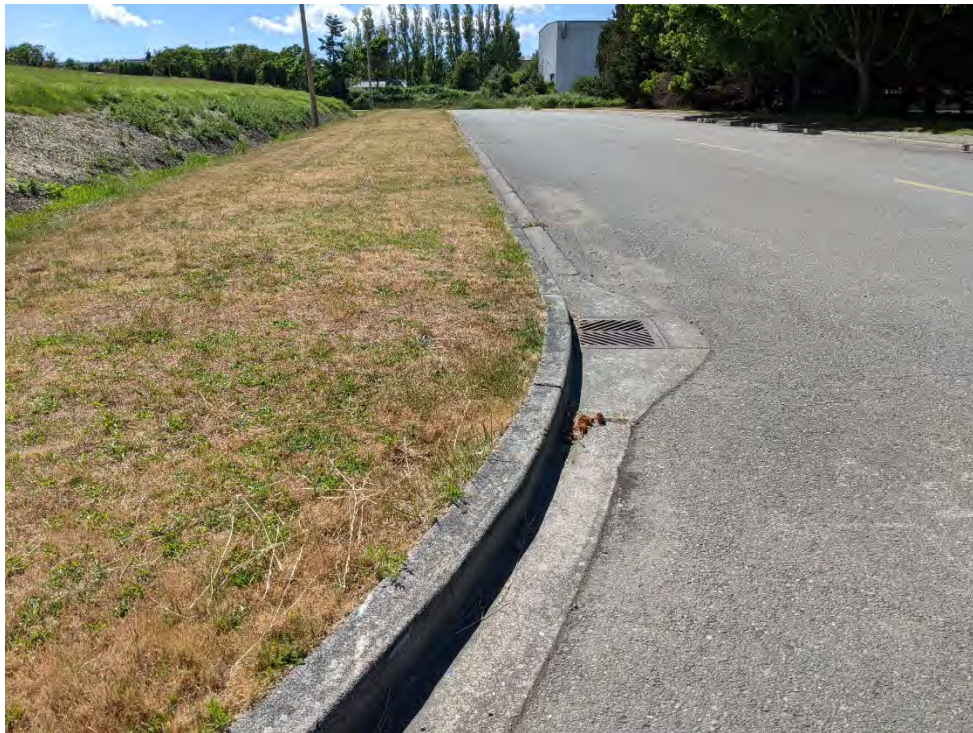
Image 6: Existing catch basin at east end of 6 th St, looking West
