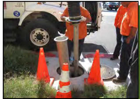
Insertion of vacuum hose into separation chamber.
