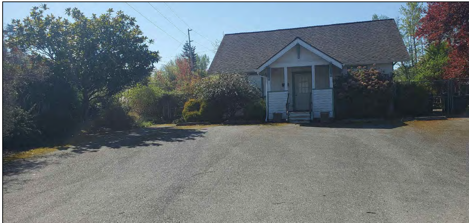
VIEW LOOKING S. 15TH STREET EXIST. RESIDENCE/PAVING TO BE REMOVED
