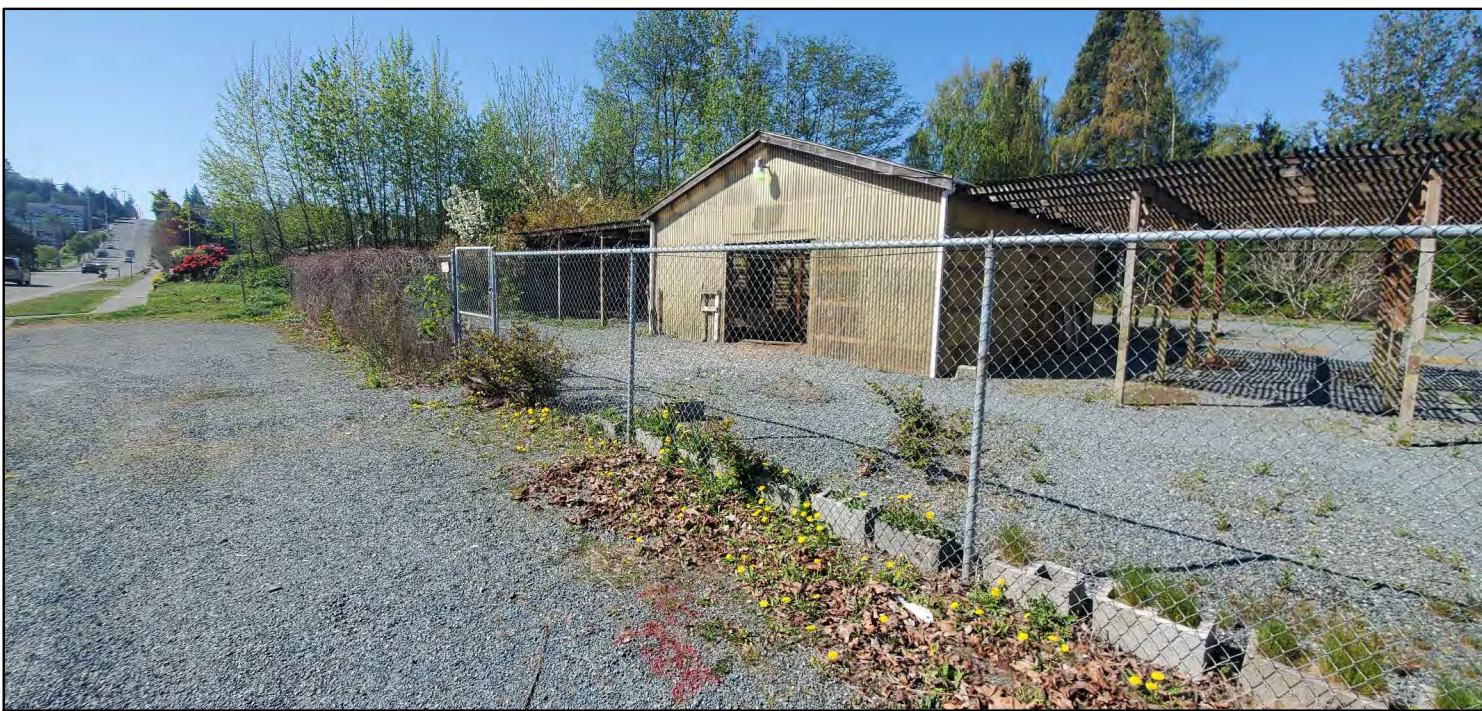
VIEW LOOKING SW FROM D AVENUE EXIST. STRUCTURE/GRAVEL TO BE REMOVED
