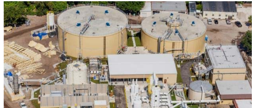
Class-A Digestion and Biogas Upgrading at the SWWRF in St. Petersburg, FL
