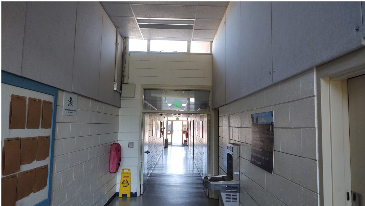
IMAGE K: EXISTING HALL, ROOM 12. LOOKING NORTH TOWARD NEW CORRIDOR, ROOM 109. EXISTING ACOUSTIC PANELS SHOWN.
