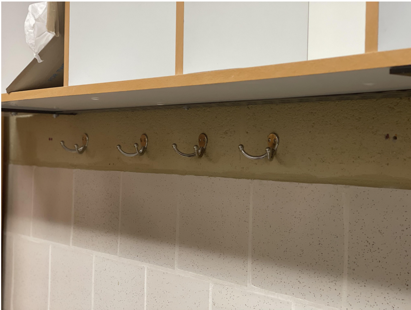
IMAGE W1: EXISTING COAT HOOKS FOR POTENTIAL SALVAGE. COORDINATE ITEMS WITH OWNER'S REPRESENTATIVE.
