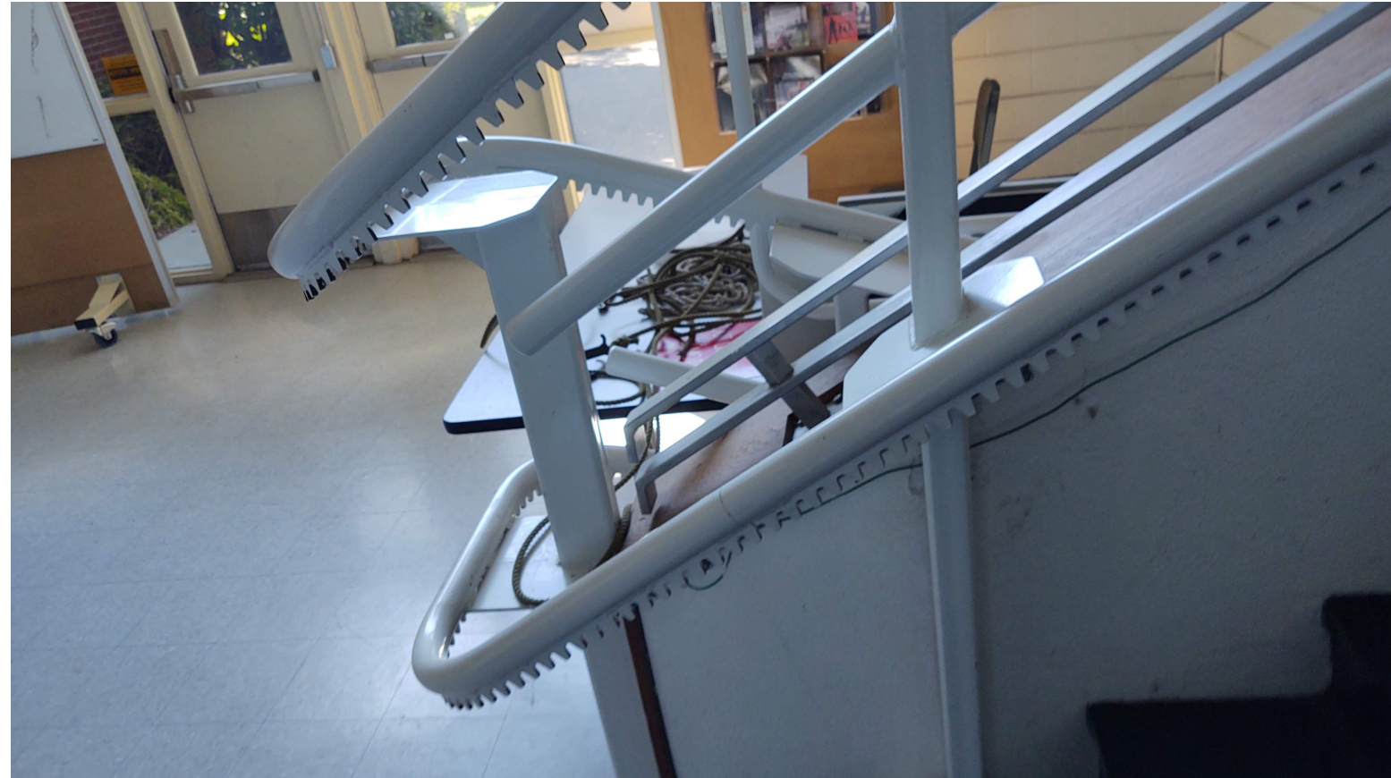
IMAGE H: EXISTING HANDRAIL AT LOBBY, ROOM 01, STAIRS.
