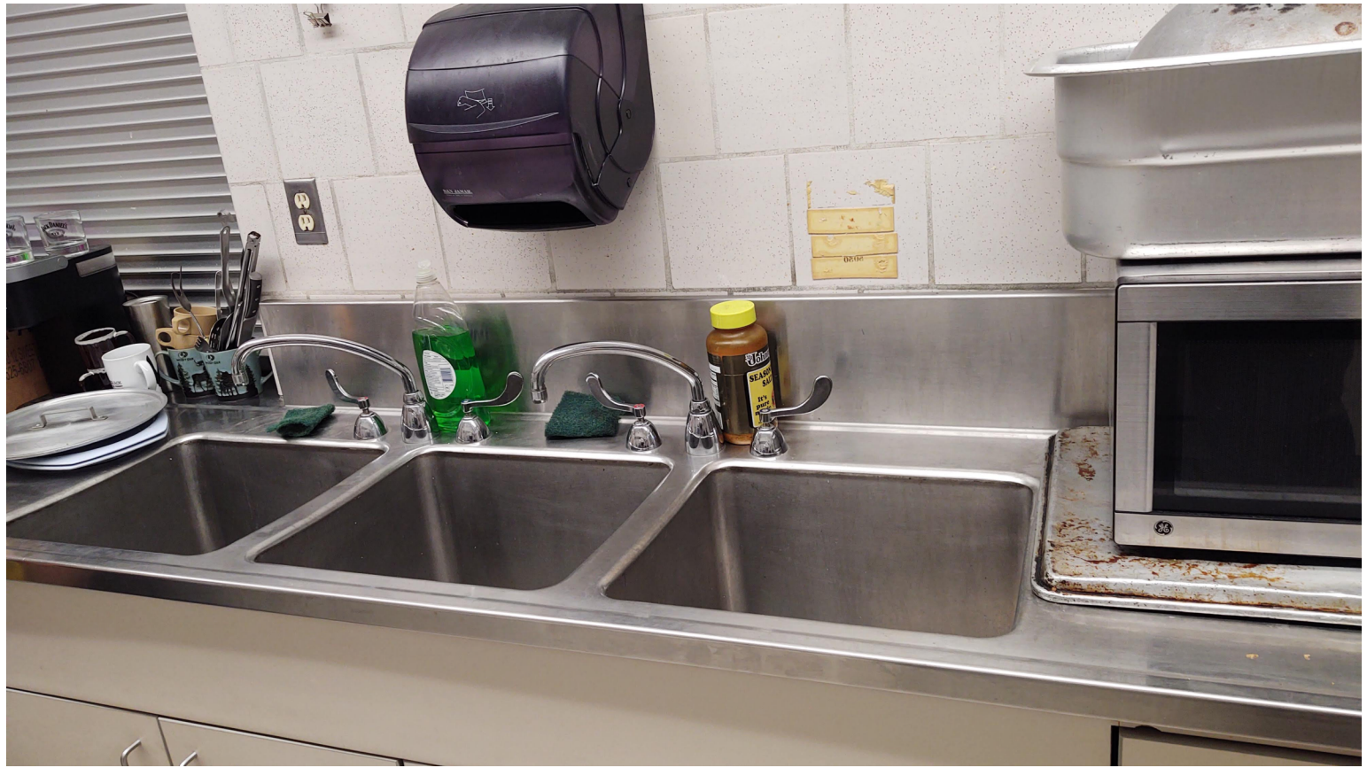
IMAGE B: EXISTING KITCHEN, ROOM 10. WEST WALL, SHOWING EXISTING CASEWORK, SINK AND OVERHEAD COILING WINDOW.
