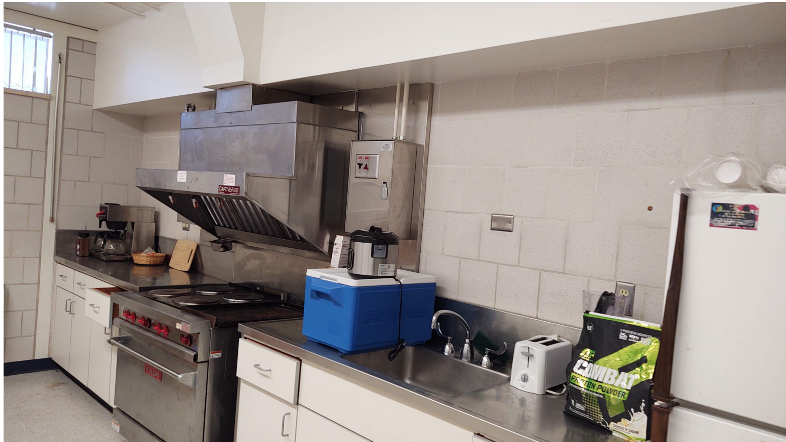
IMAGE A: EXISTING KITCHEN, ROOM 10. EAST WALL, SHOWING EXISTING COMMERCIAL RANGE AND HOOD, EXISTING CASEWORK, SOFFIT AND REFRIGERATOR.
