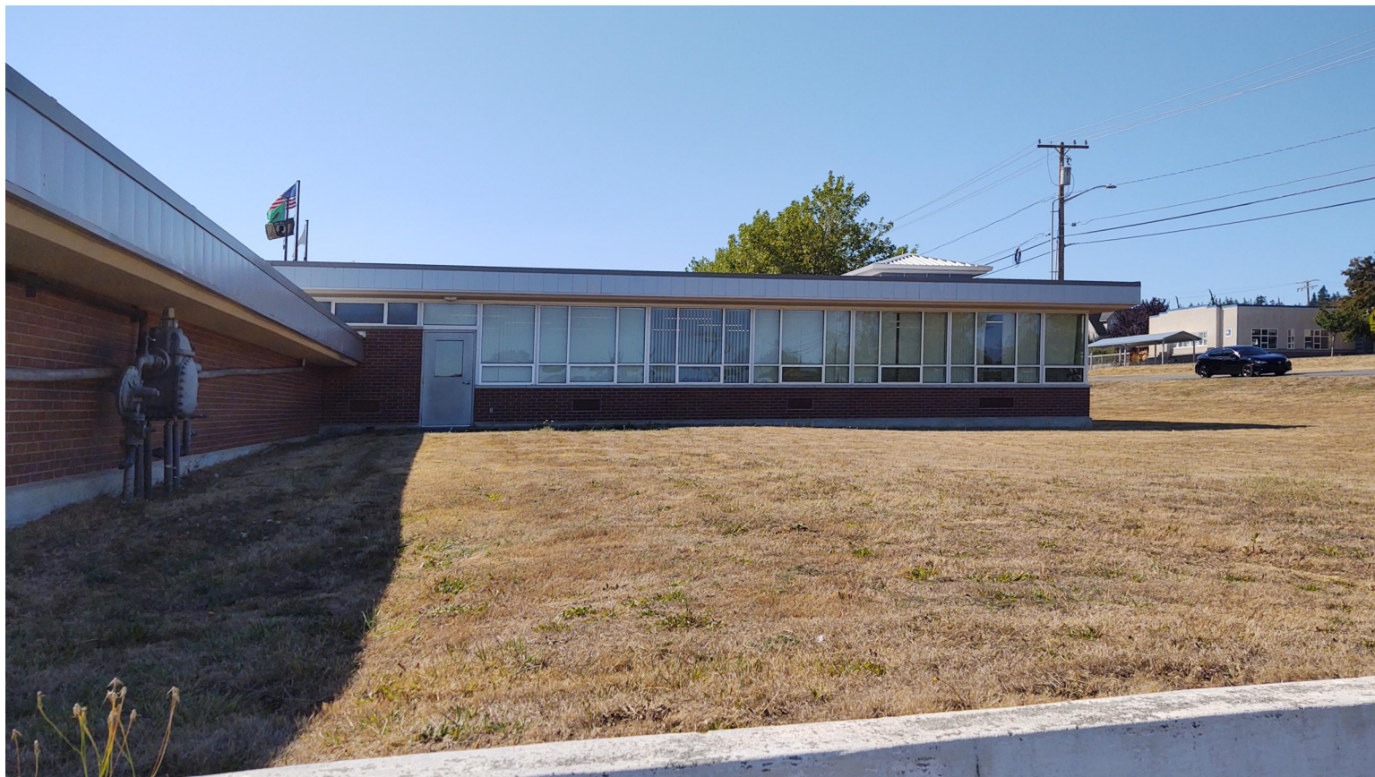
IMAGE Q: EXTERIOR OF EXISTING OPEN OFFICE WING, ROOM 08, AT RETAINING WALL LOOKING SOUTH WEST.
