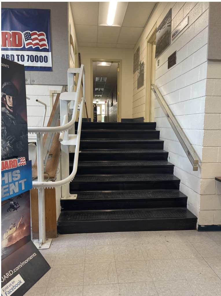
IMAGE Y: EXISTING HANDRAILS. LOBBY, ROOM 01, STAIRS.
