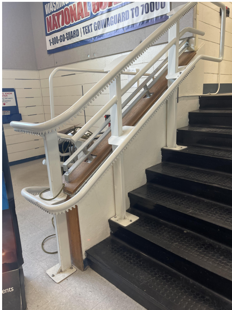
IMAGE Y1: EXISTING STEEL POST AND TRACK FOR EXISTING CHAIR LIFT, AND EXISTING ALUMINUM HANDRAIL ATTACHED TO WOOD VENEERED CONCRETE WALL.
