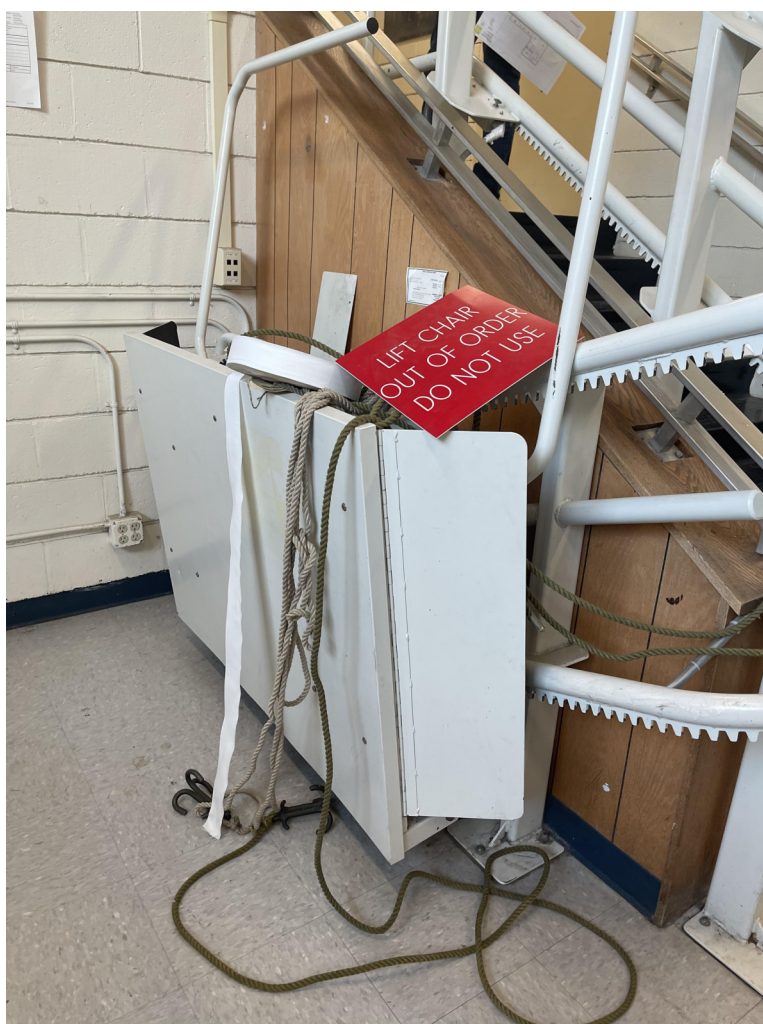
IMAGE Y2: EXISTING ADA LIFT AND HANDRAILS. LOBBY, ROOM 01.
