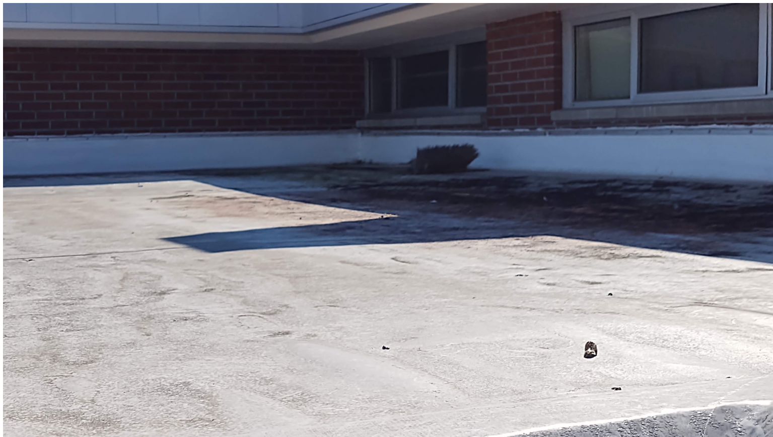
IMAGE T: EXISTING ROOF.
