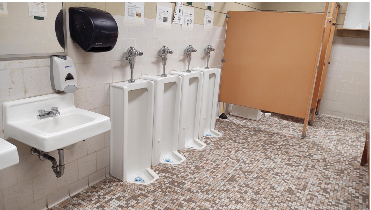
IMAGE C: EXISTING MEN'S RESTROOM, ROOM 20. NORTH WALL, SHOWING EXISTING SINKS, URINALS, METAL PARTITIONS, WALL TILING AND MOSAIC TILE FLOORING . TYPICAL RESTROOM FINISH AND FIXTURE CONDITIONS.
