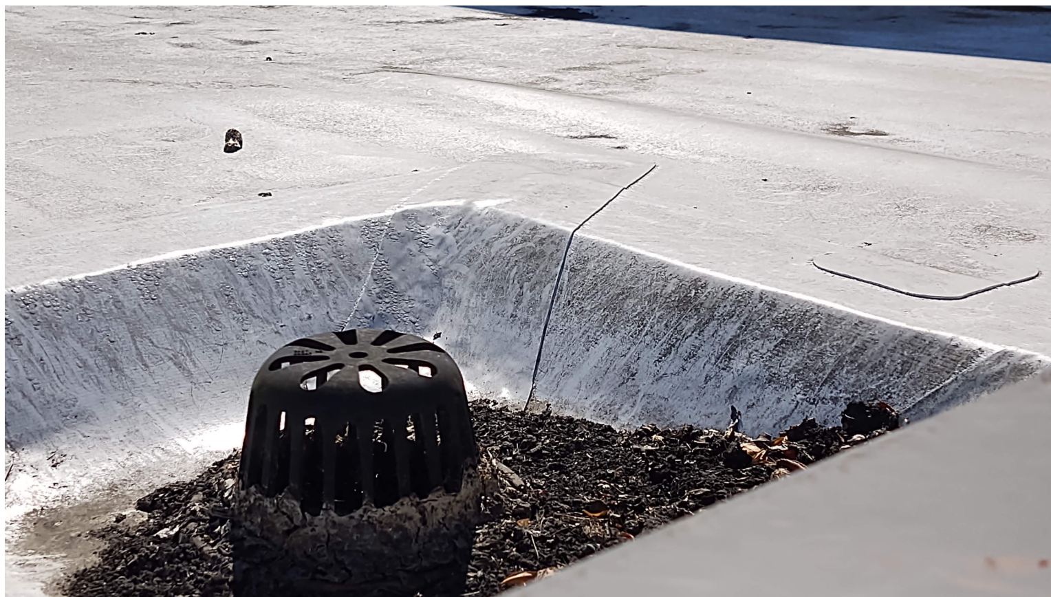
IMAGE V: EXISTING ROOF DRAIN.
