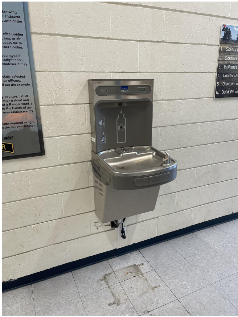
IMAGE X: EXISTING DRINKING FOUNTAIN FOR POTENTIAL SALVAGE. COORDINATE ITEMS WITH OWNER'S REPRESENTATIVE.
