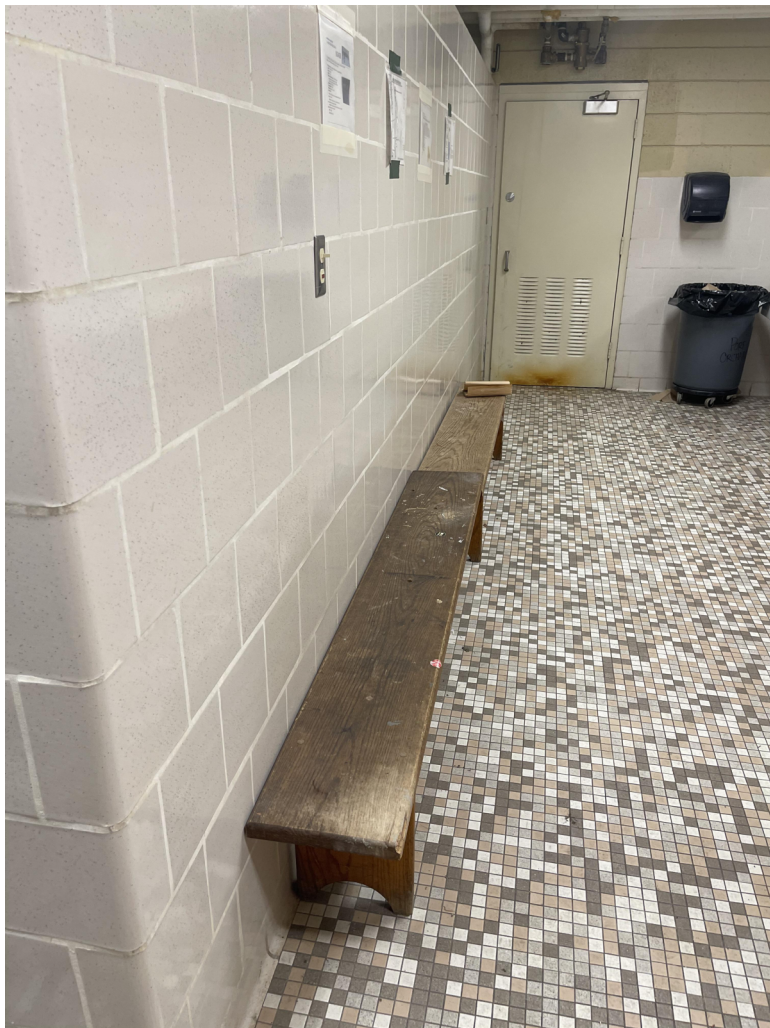
IMAGE W2: EXISTING SHOWER ROOM BENCHES FOR POTENTIAL SALVAGE. COORDINATE ITEMS WITH OWNER'S REPRESENTATIVE.
