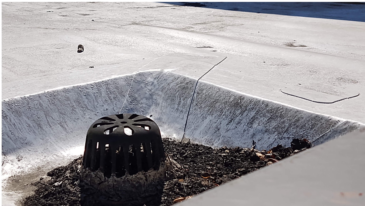
IMAGE V: EXISTING ROOF DRAIN.
