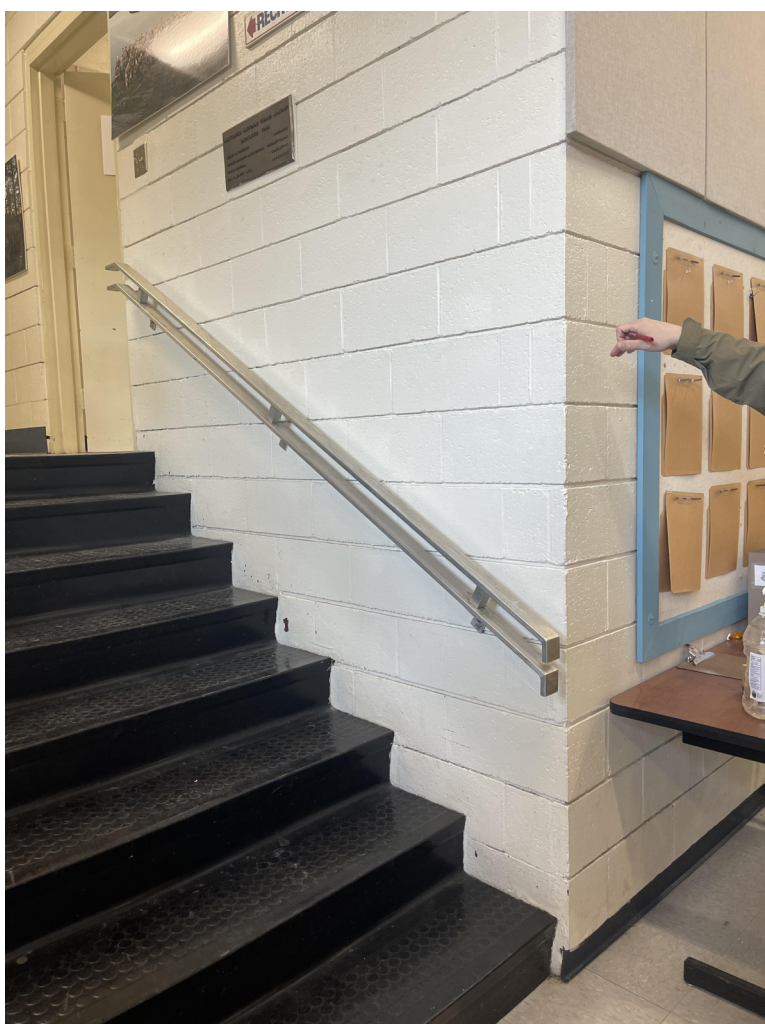
IMAGE Y3: EXISTING ALUMINUM HANDRAIL ATTACHED TO EXISTING CMU WALL WITH 3 WALL BRACKETS.
