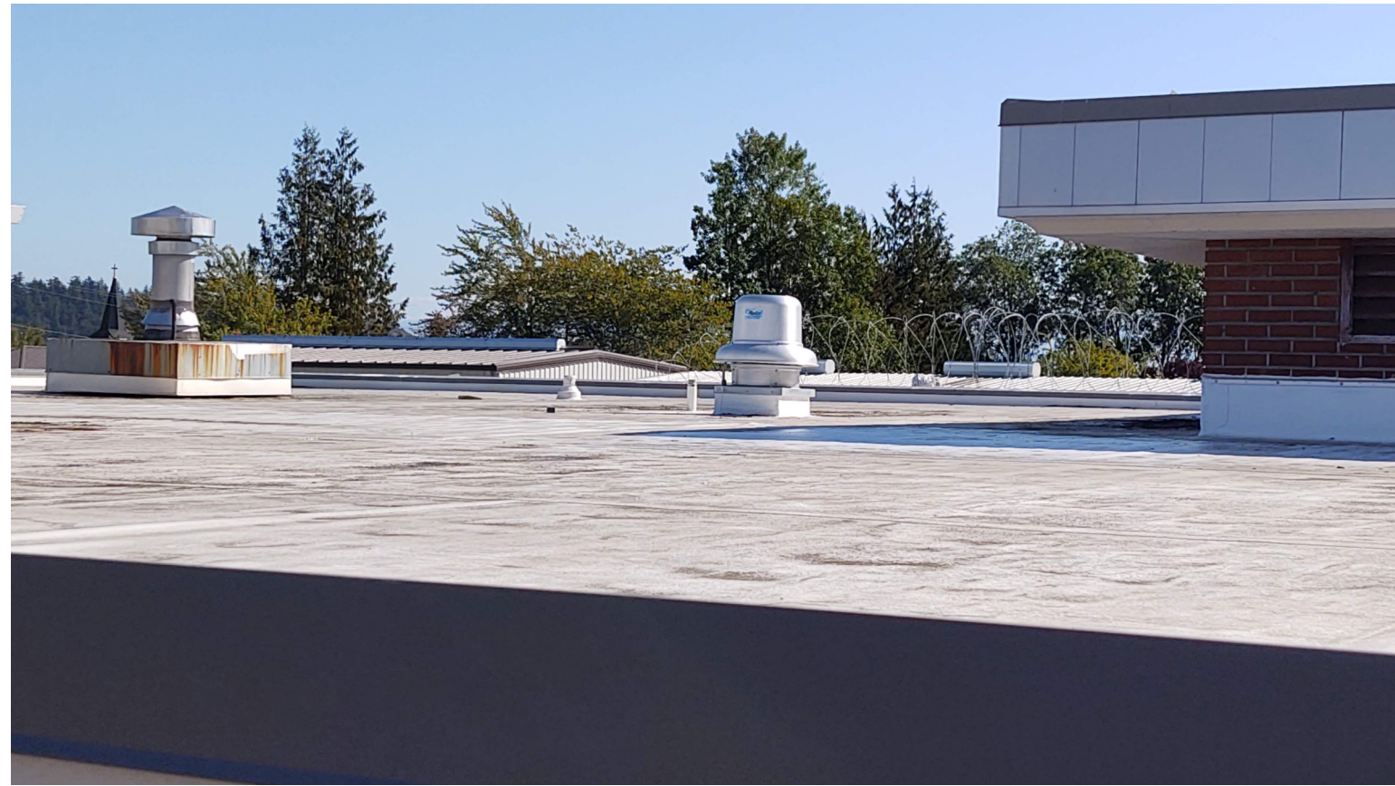
IMAGE S: EXISTING ROOF LOOKING NORTH EAST
