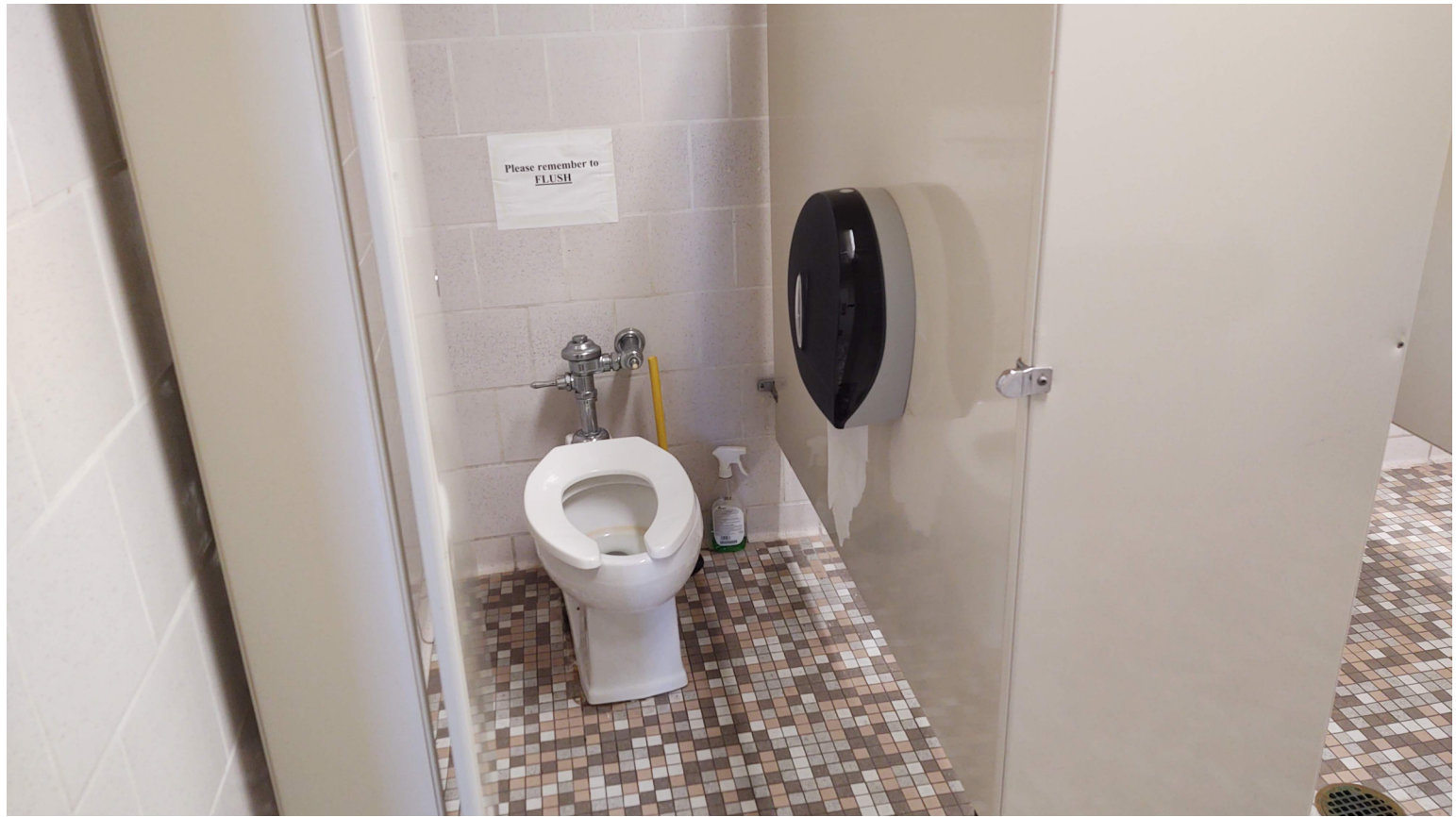
IMAGE D: EXISTING FLOOR MOUNTED TOILET FIXTURE (TYPICAL) AND METAL PARTITIONS.
