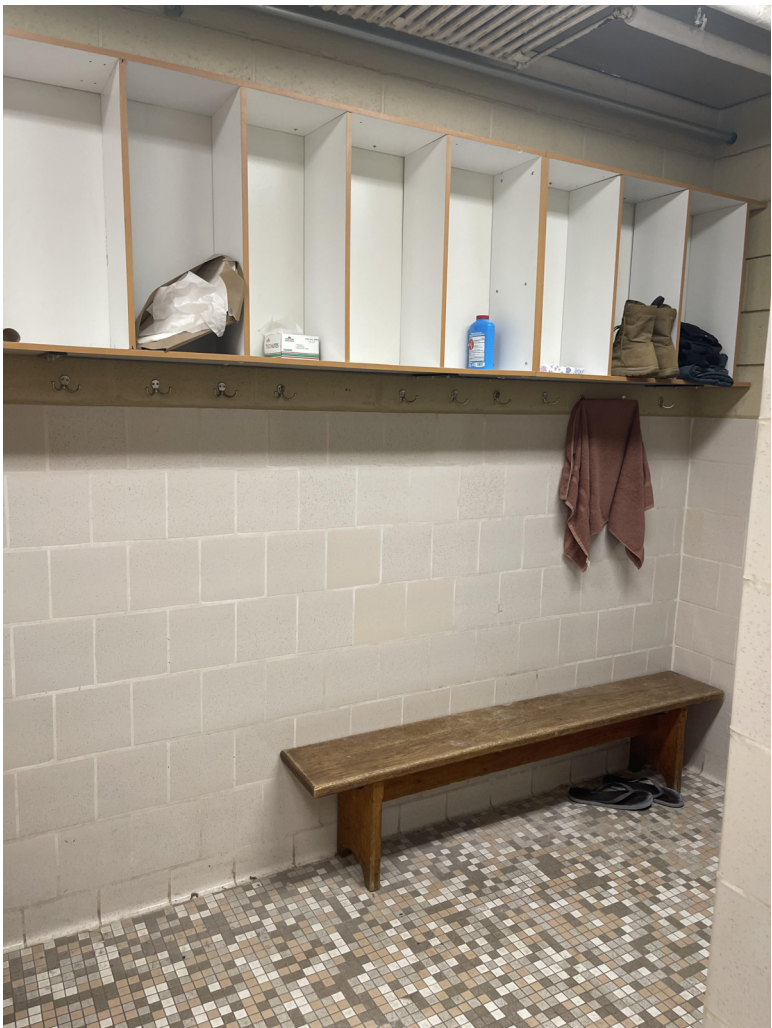
IMAGE W: EXISTING BENCH, CASEWORK AND COAT HOOKS FOR POTENTIAL SALVAGE. COORDINATE ITEMS WITH OWNER'S REPRESENTATIVE.
