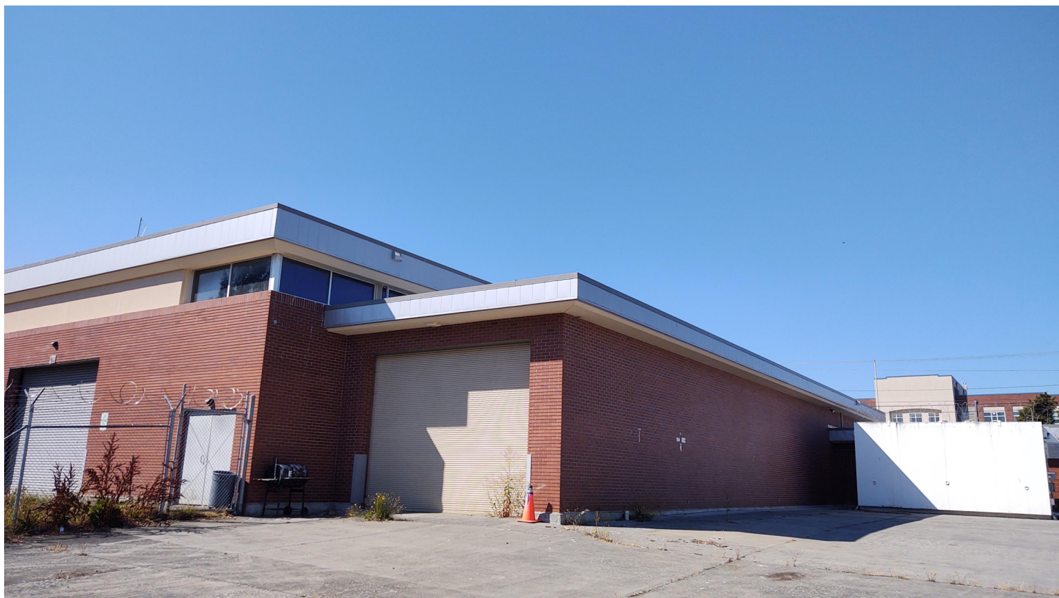
IMAGE R: EXISTING DRILL HALL, ROOM 22 AND STORAGE, ROOM 23D. LOOKING SOUTH WEST AT EXTERIOR BRICK WALL AT LOCATION OF NEW CLASSROOMS.
