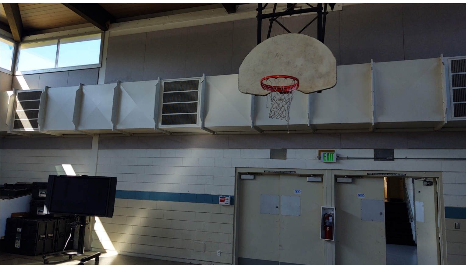
IMAGE N: EXISTING DRILL HALL, ROOM 22. LOOKING WEST AT EXISTING DUCT WORK AND ACOUSTIC PANELS.
