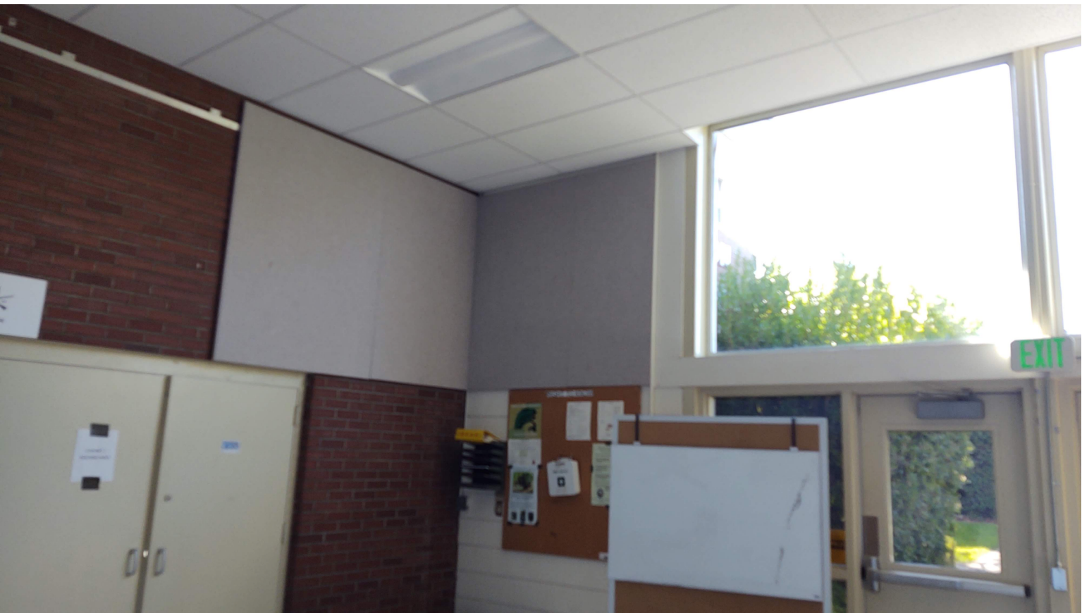
IMAGE M: EXISTING LOBBY, ROOM 01. LOOKING SOUTH EAST AT EXISTING ACOUSTIC PANELS.
