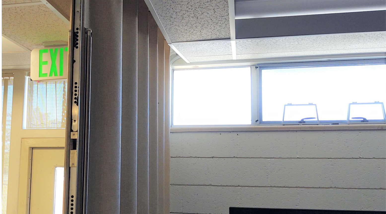
IMAGE F: EXISTING OPEN OFFICE, ROOM 08. TYPICAL CLERESTORY WINDOW, ROOM DIVIDER AND CEILING CONDITIONS SHOWN.
