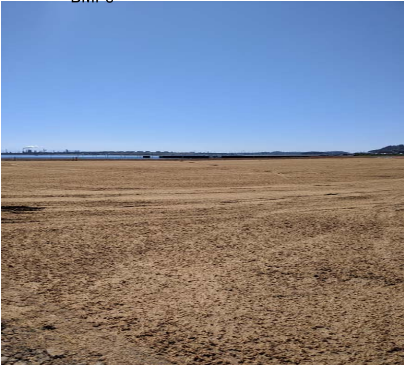
Site grading and BMPs
