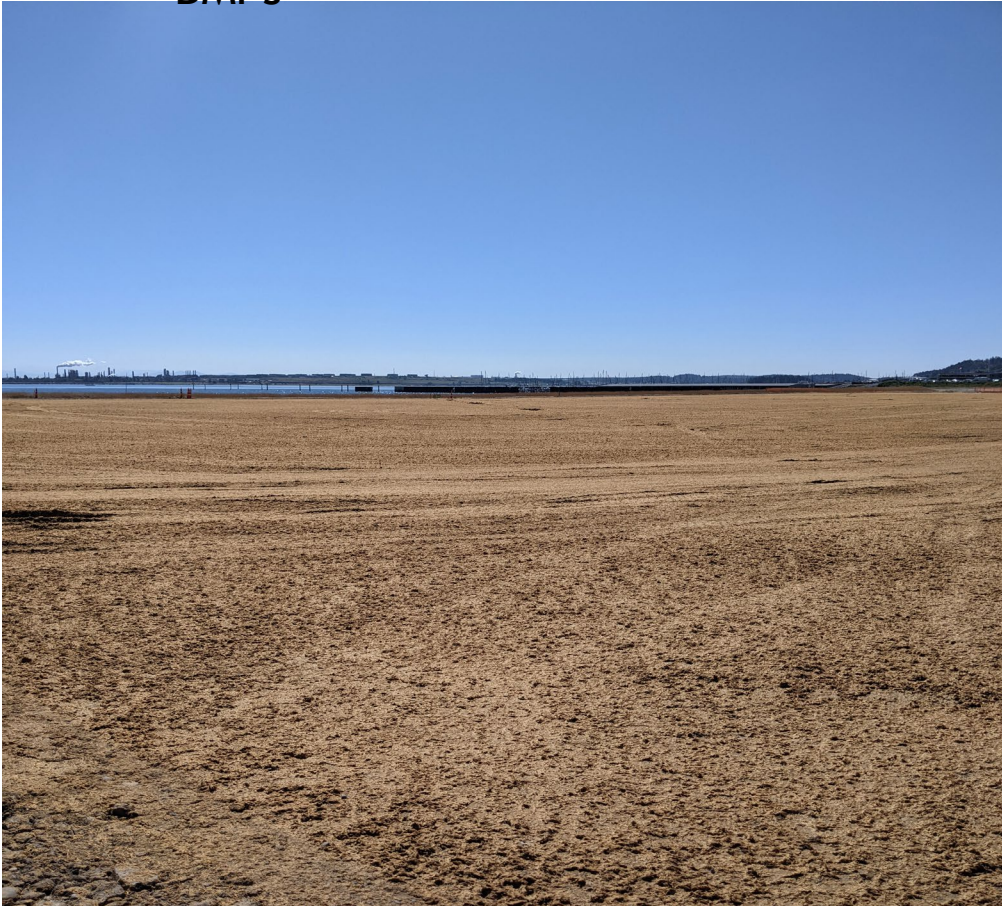
Site grading and BMPs
