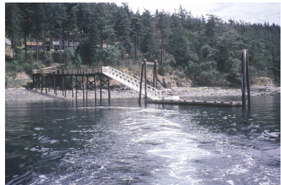
Fig. 1 – A typical pier, ramp, and float arrangement used for residential boat moorage in Puget Sound, Washington.
