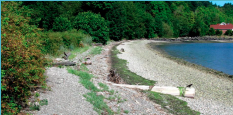
Soft shoreline project in Anacortes, Washington, uses logs and beach nourishment instead of rock and concrete. Photo credit: Hugh Shipman.
