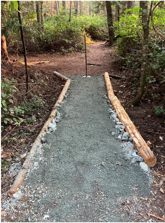
New turnpike, Clyde Way Trail 109 access. MacLeod tool for scale.
