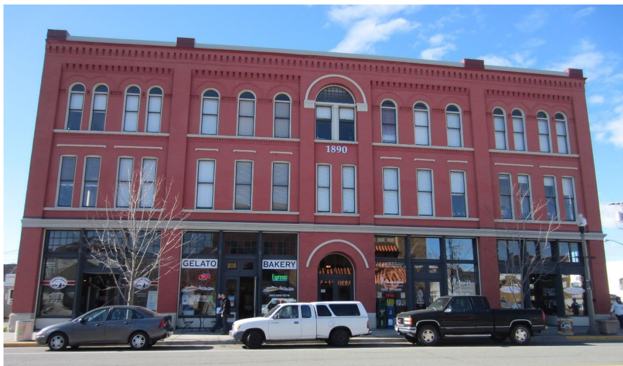
Figure 8 - The historic Wilson Hotel building
