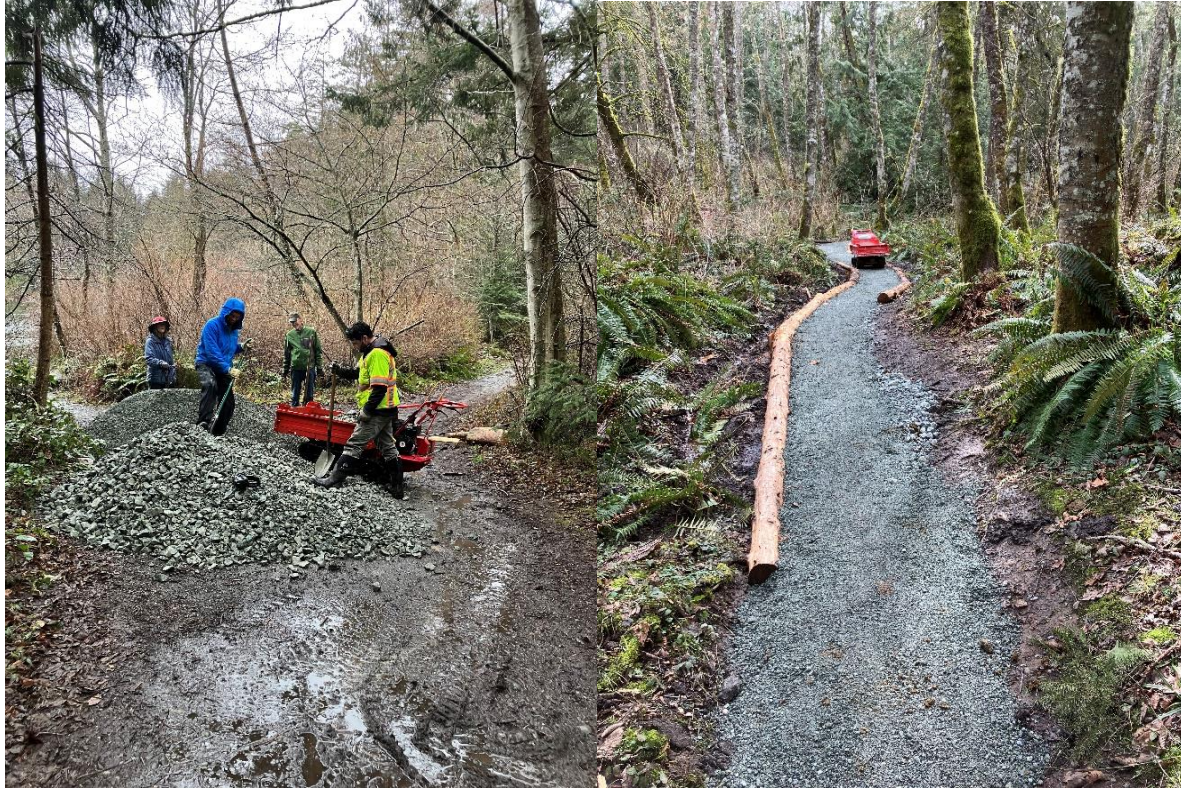
3/4/23: Volunteers help Braydn Krueger to load the power wheelbarrow for resurfacing work on Trail 224; the final product.
