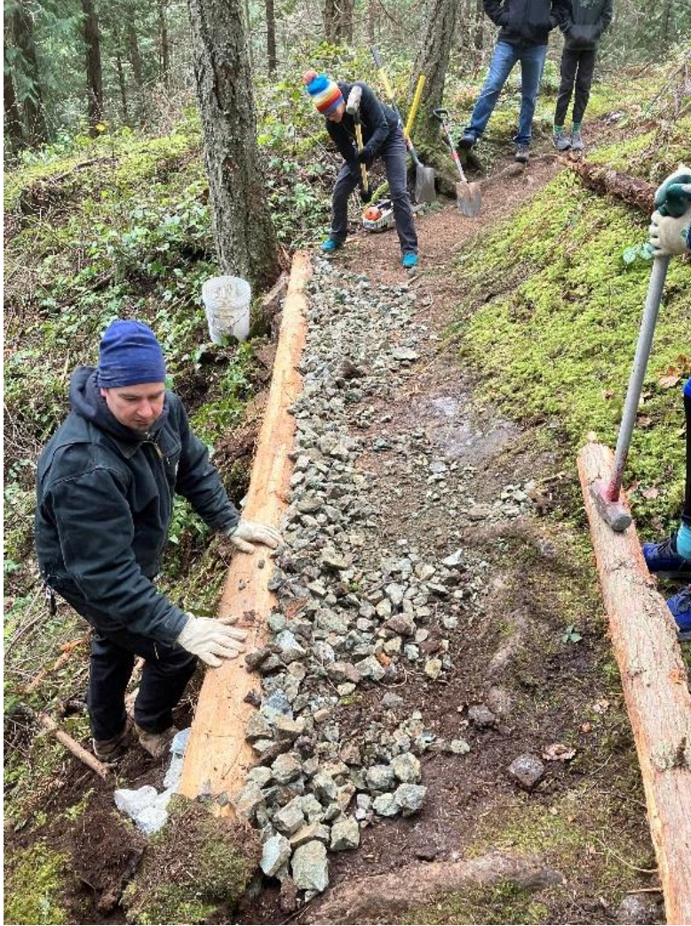
2/25/23: Fidalgo Trail Riders volunteers replacing one of two degraded turnpikes on Trail 220 and resurfacing the trail.
