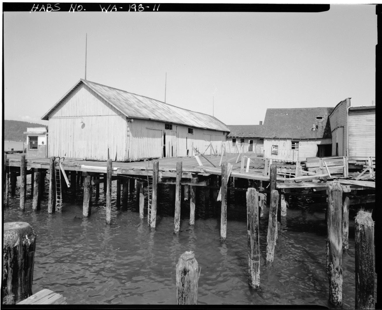
Photocopy of photograph (Original print, Port of Anacortes.) Brady's Anacortes Studio, Photographer, date unknown. Overview of Curtis Wharf. North section of main dock is intact; Sand and Gravel Wharf on the right. - Curtis Wharf, O & Second Streets, Anacortes, Skagit County, WA
