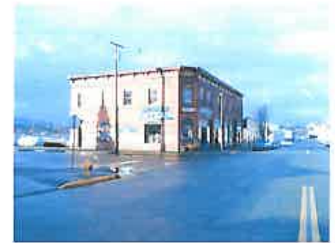
Figure 49. Northwest Corner of 3rd Street and Commercial Avenue
