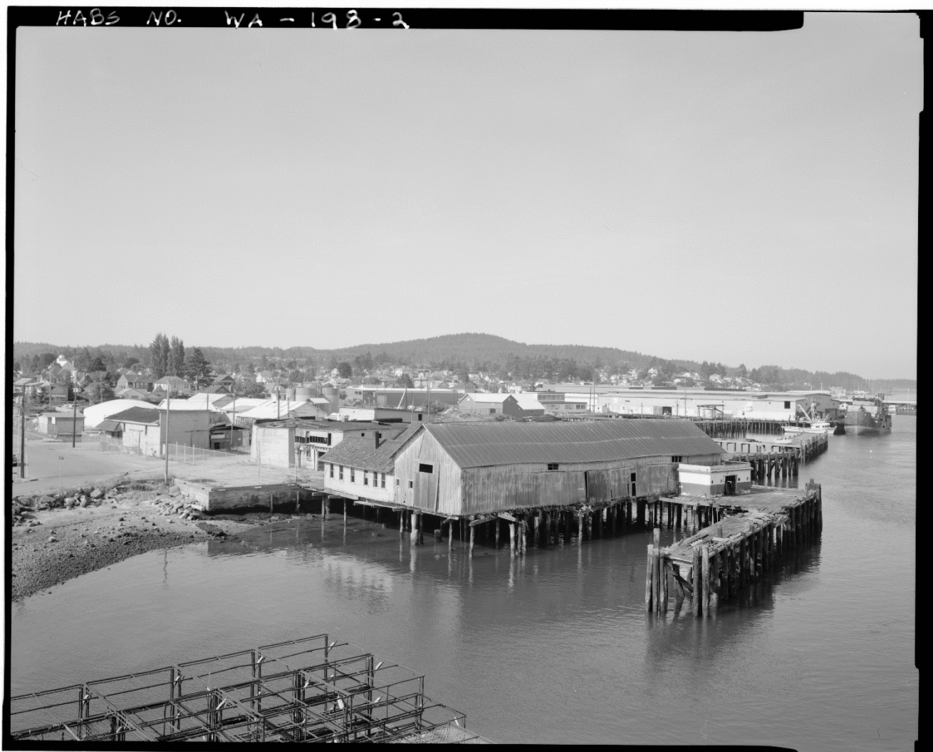
Panoramic view, Curtis Wharf, from the top of a tanker barge at the Port of Anacortes. View looking south. - Curtis Wharf, O & Second Streets, Anacortes, Skagit County, WA
