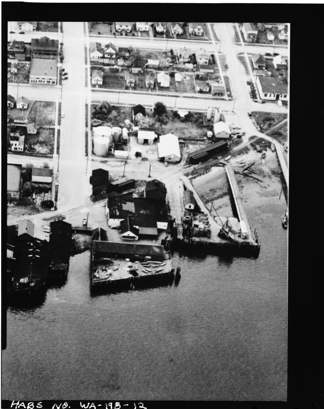
Photocopy of photograph (Original print, Port of Anacortes.) Brady's Anacortes Studio, Photographer, date unknown. Overview of Curtis Wharf and surrounding area. North section of main dock is intact; Sand and Gravel Wharf on the right. - Curtis Wharf, O & Second Streets, Anacortes, Skagit County, WA
