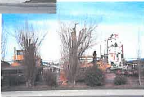
Figure 35. Sparse Planting along the Pier 2 Fence Line
