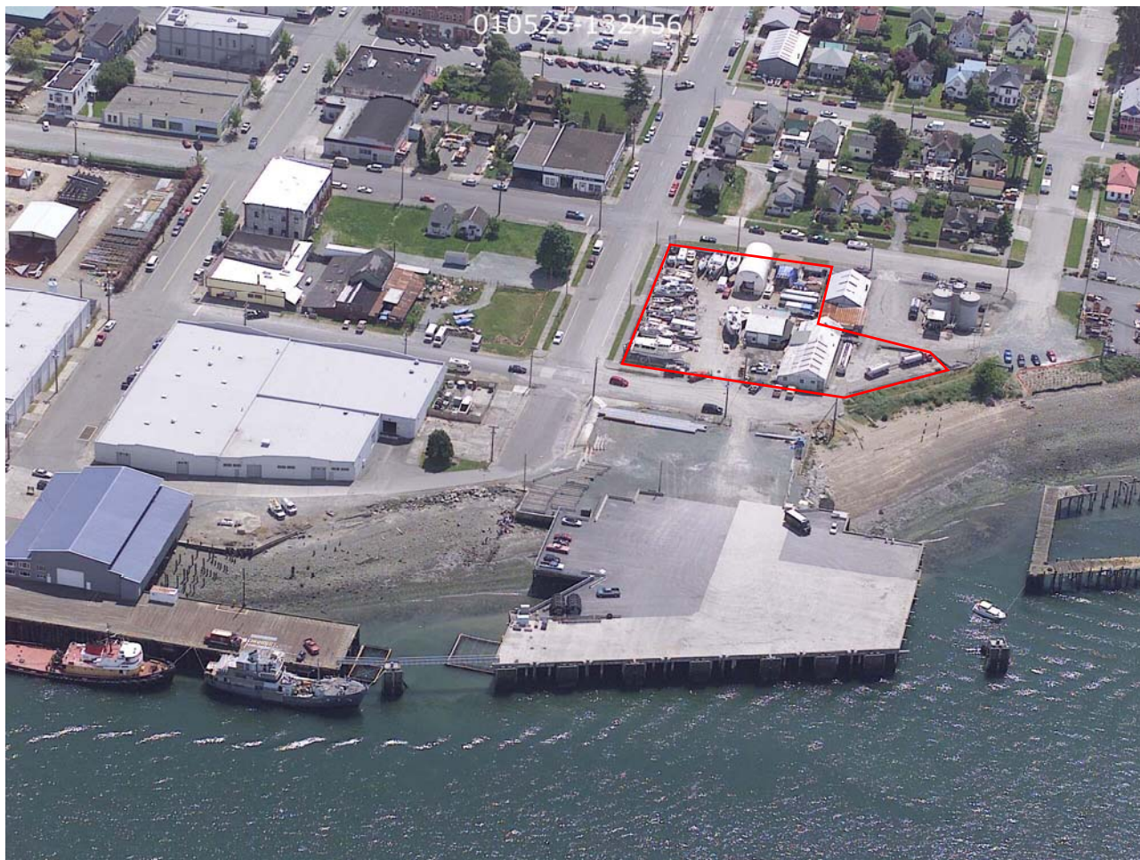
Overview of Quiet Cove and surrounding area - O & Second Streets, Anacortes, Skagit County, WA
