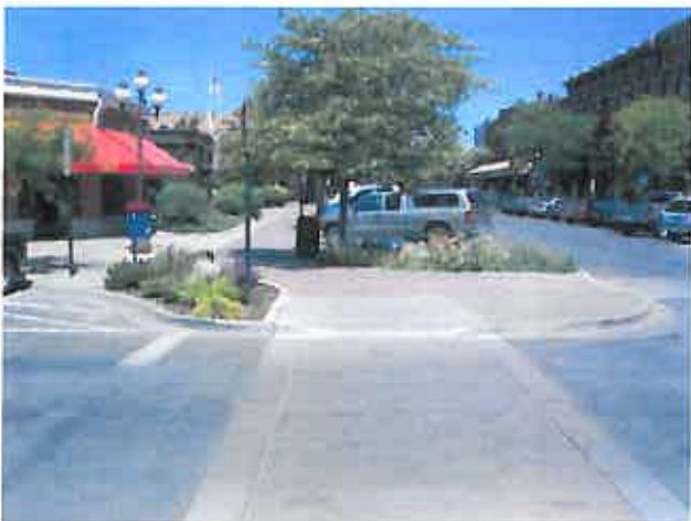
Curb bulbs at street intersections and specially paved crosswalks can provide a safe and comfortable walking environment for pedestrians.
