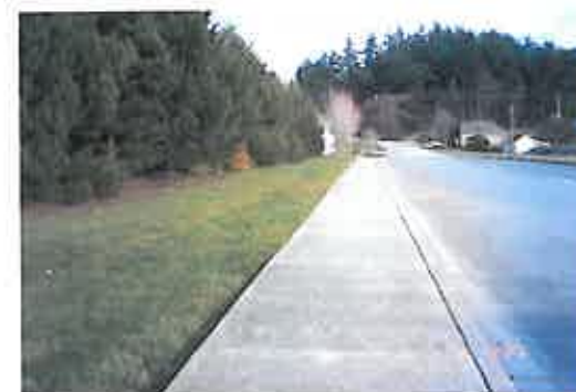
Figure 30. Existing Sidewalk on 6th Street
