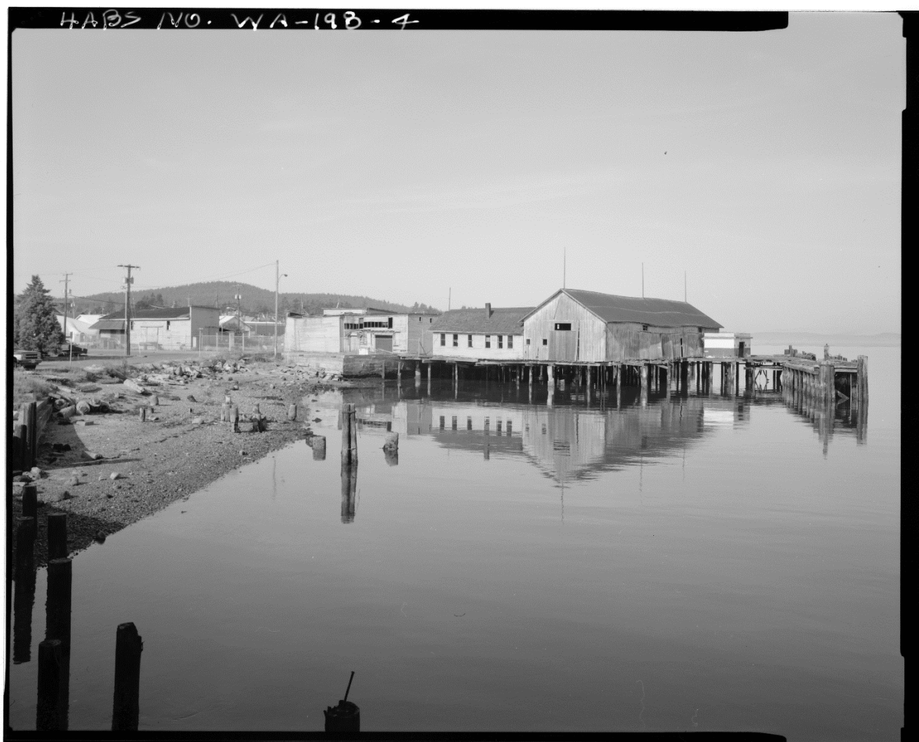
East side of Curtis Wharf, as seen from the pier at the Port of Anacortes. View looking south and west. - Curtis Wharf, O & Second Streets, Anacortes, Skagit County, WA
