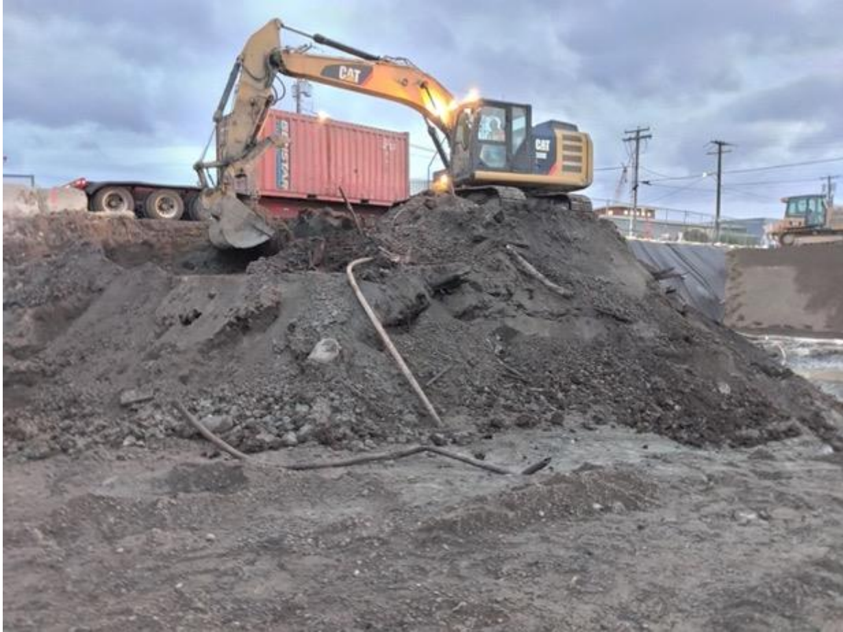
Figure 147. Small portion of fill to be removed.
