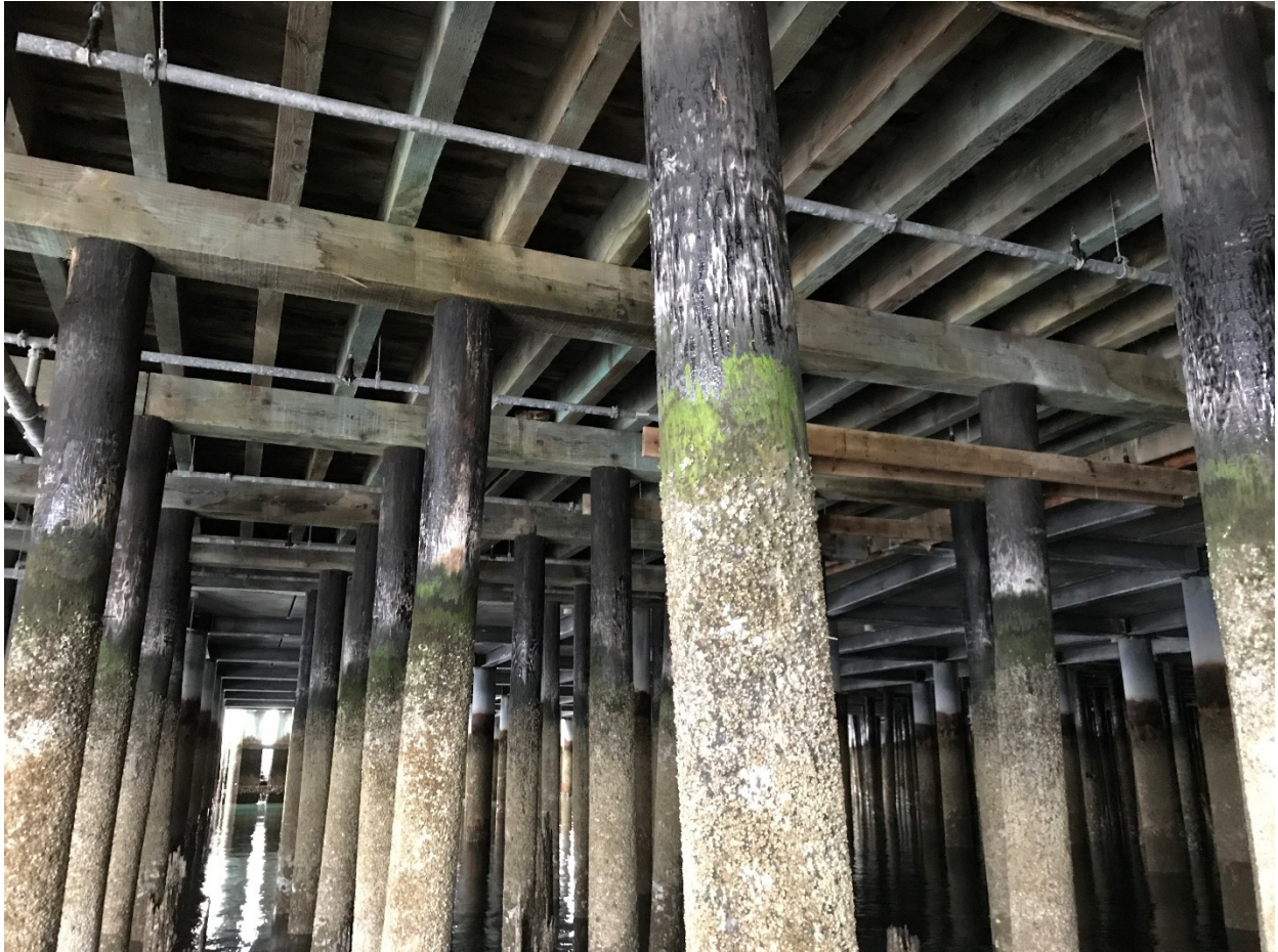
Under-wharf view from the bulkhead looking north. Pipe is for fire suppression system.
