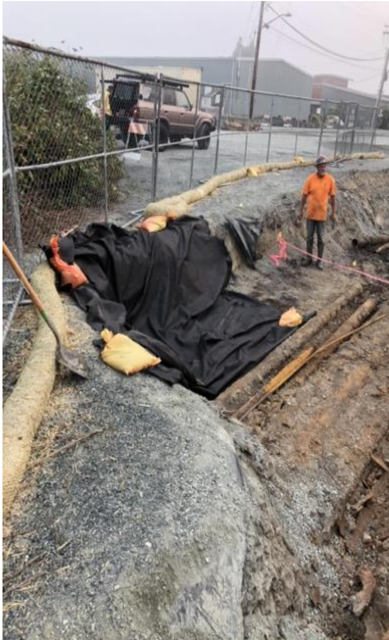
Figure 63. Covering shell midden with geotextile fabric.
