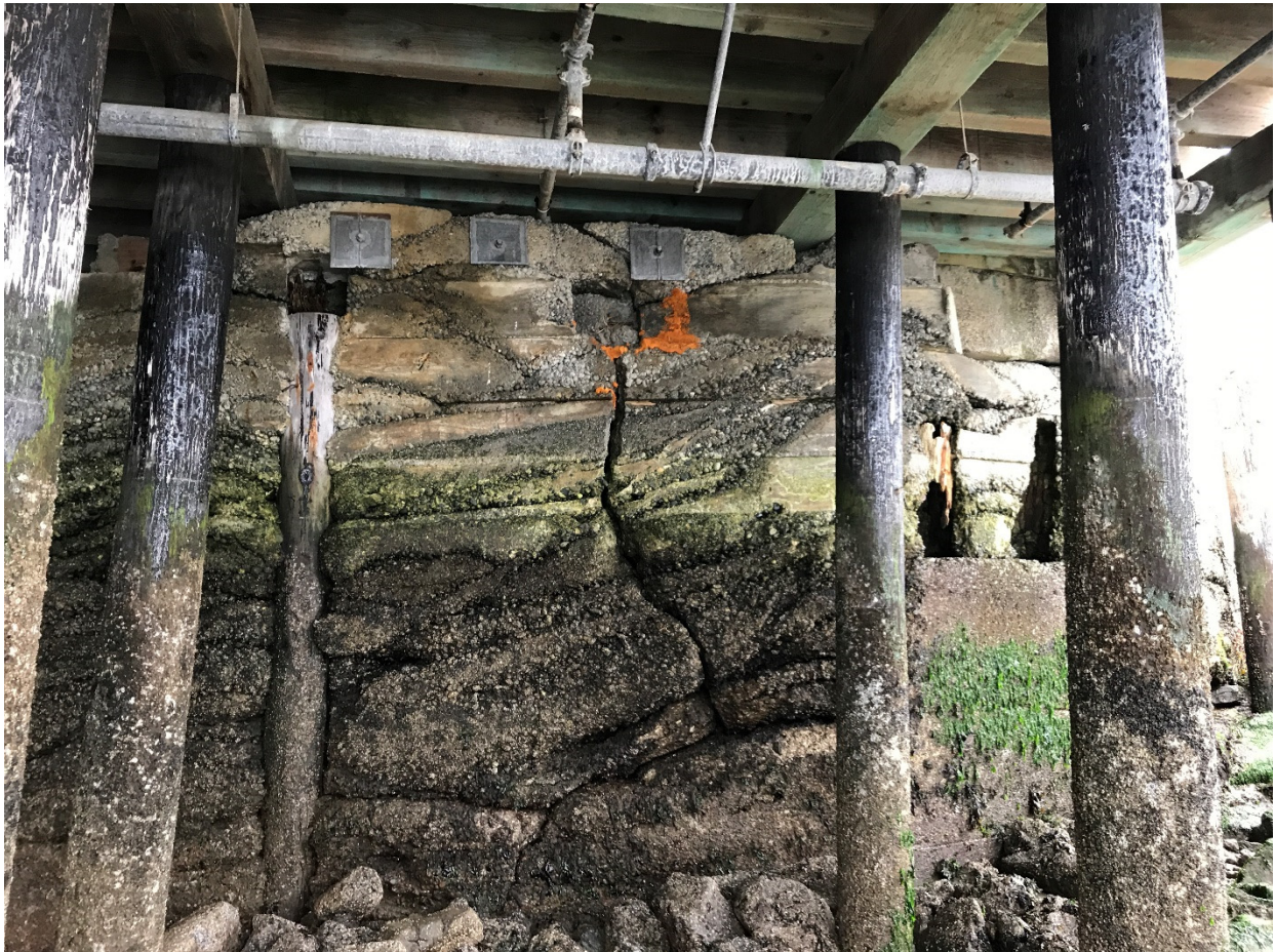
Under-wharf view of the southwest bulkhead on Curtis Wharf. Pipe is for fire suppression system. No evidence of historical product lines coming through the bulkhead.
