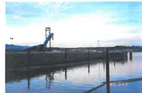
Figure 43. View of Pier 2 from "T" Avenue
