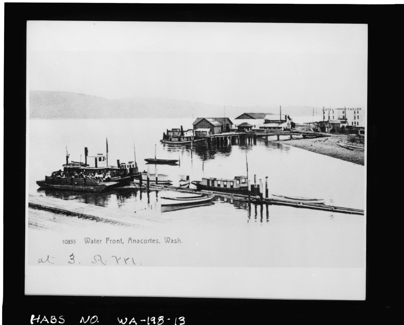
Photocopy of photograph (Original print, Anacortes Museum.) Photographer unknown. Early view, c. 1905, looking north and east, before the construction of the Cement and Plaster Warehouse and the expansion of the wharf itself to the west. - Curtis Wharf, O & Second Streets, Anacortes, Skagit County, WA
