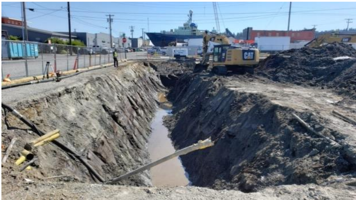
Figure 13. Extent of excavations, facing East from driveway at Western edge of project. Pipe platform visible on right side of photo.
