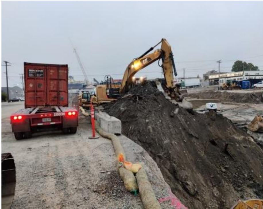
Figure 139. Overview of progress near end of project.
