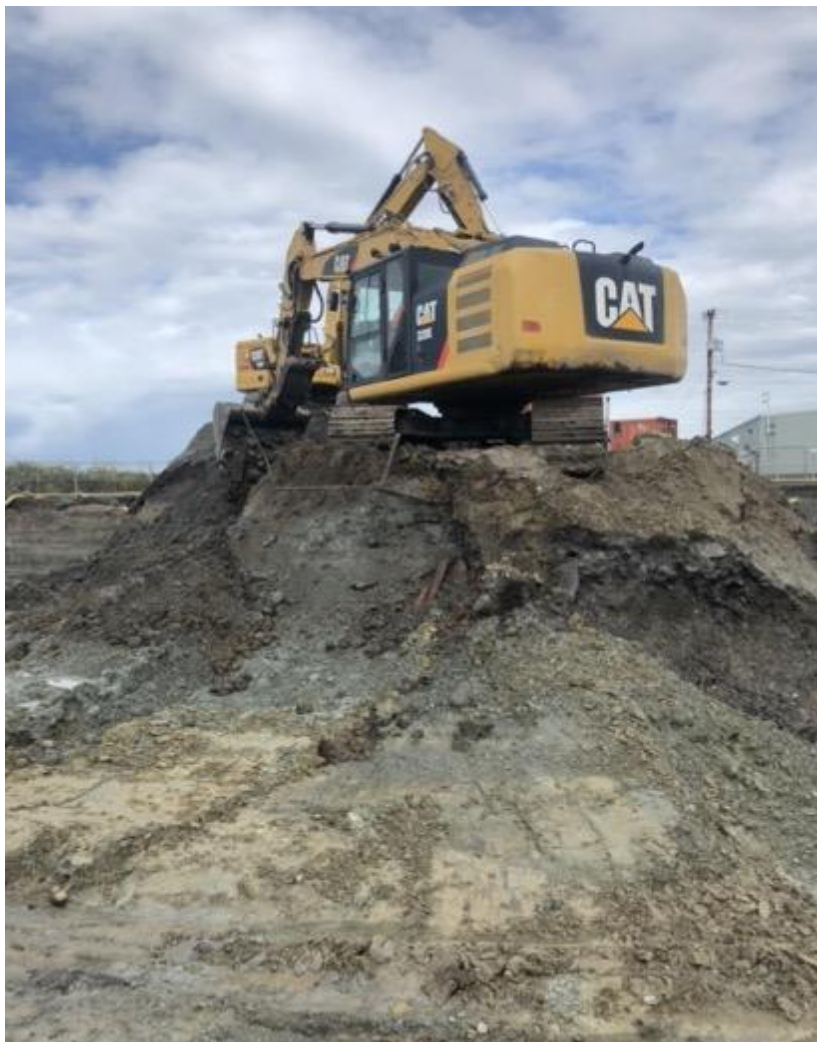
Figure 123. Photo taken facing West, showing the excavation progress at southern edge of the site.
