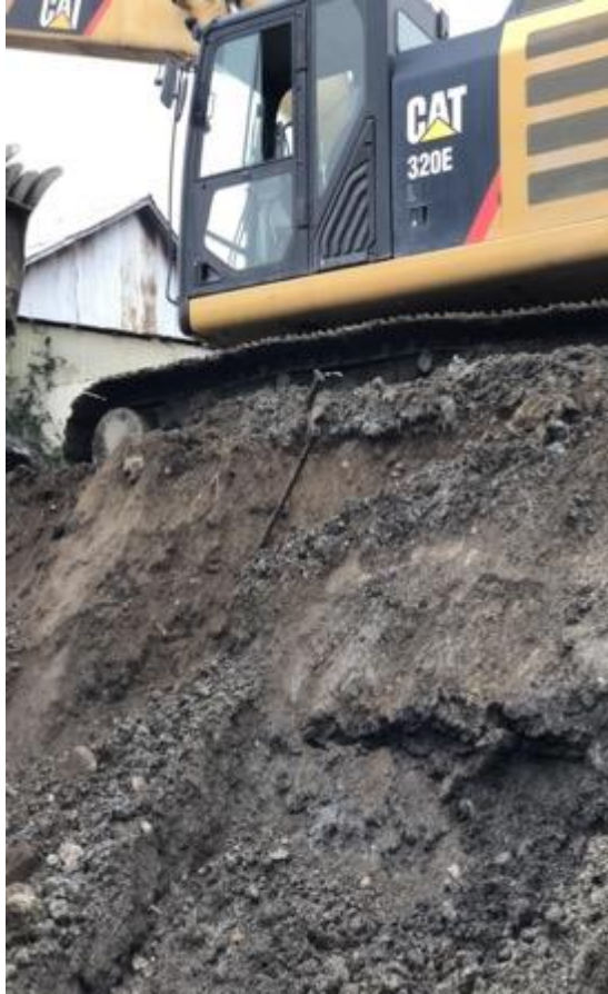
Figure 76. Photo taken facing Southwest of the excavator on the temporary road; showing in situ modern metal piping likely from plumbing in the building which used to stand there.
