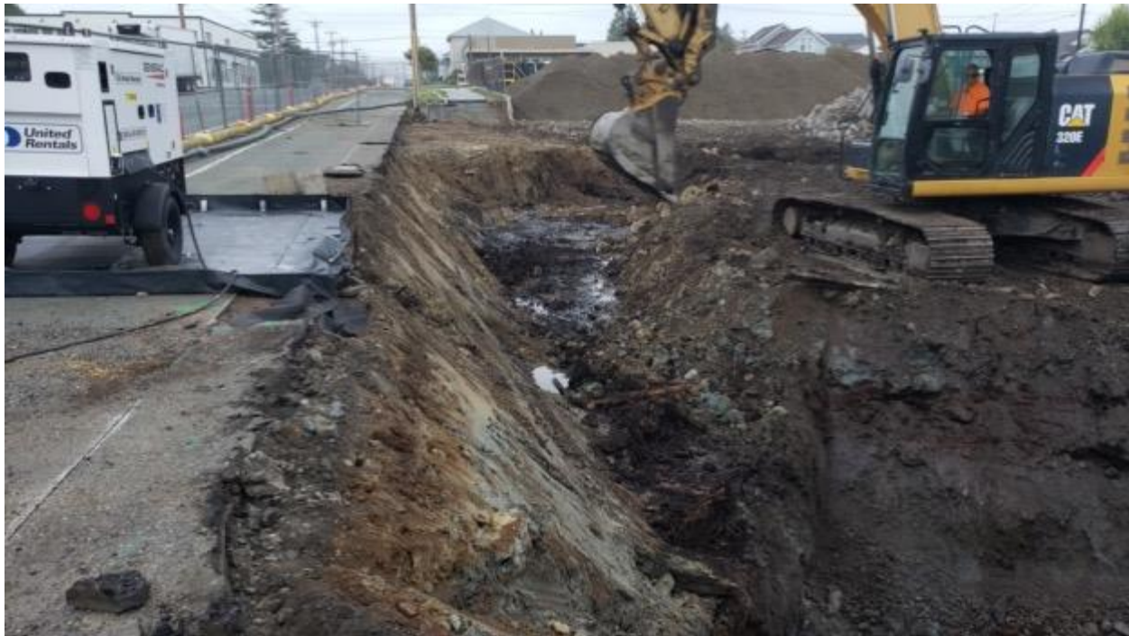
Figure 16. Start of day site overview, facing South from NE corner of project
