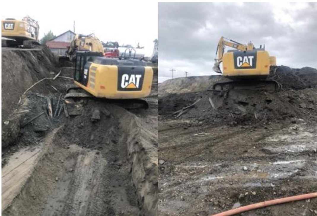
Figure 111. Left: facing south shot of the excavation observed today. Right: the CAT excavator sitting on what was the coal shed.
