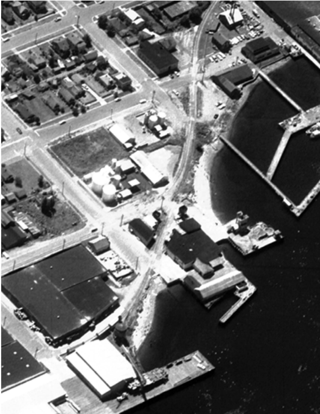
Overview of Quiet Cove and surrounding area. Reisner Petroleum Terminal to the south of Curtis Wharf is intact; Standard Oil Facility and railroad line in central portion of photograph. - O & Second Streets, Anacortes, Skagit County, WA
