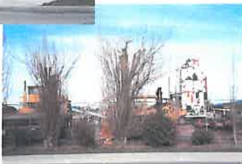
Figure 35. Sparse Planting along the Pier 2 Fence Line
