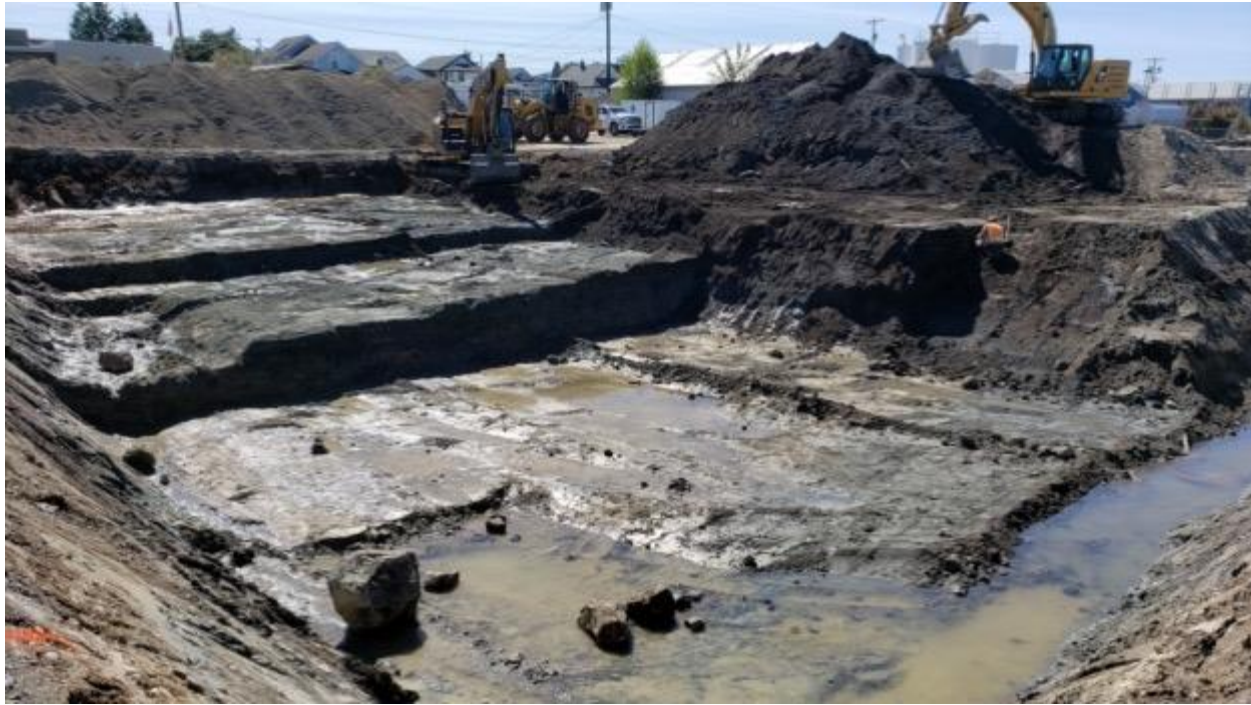
Figure 39. End of day overview, looking SSW from NE corner
