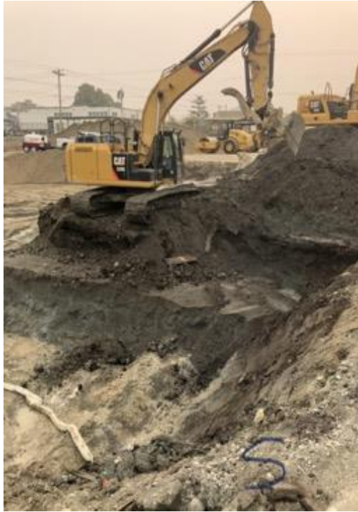
Figure 55. The site about midway through the day (facing SE) showing the excavator machine and the progress of the dig.
