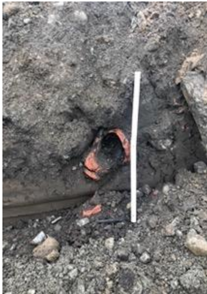
Figure 77. Intact terra cotta ceramic sewage pipe in situ on the southern wall of the excavation (in the eastern side of the site) photo taken facing south towards scale.
