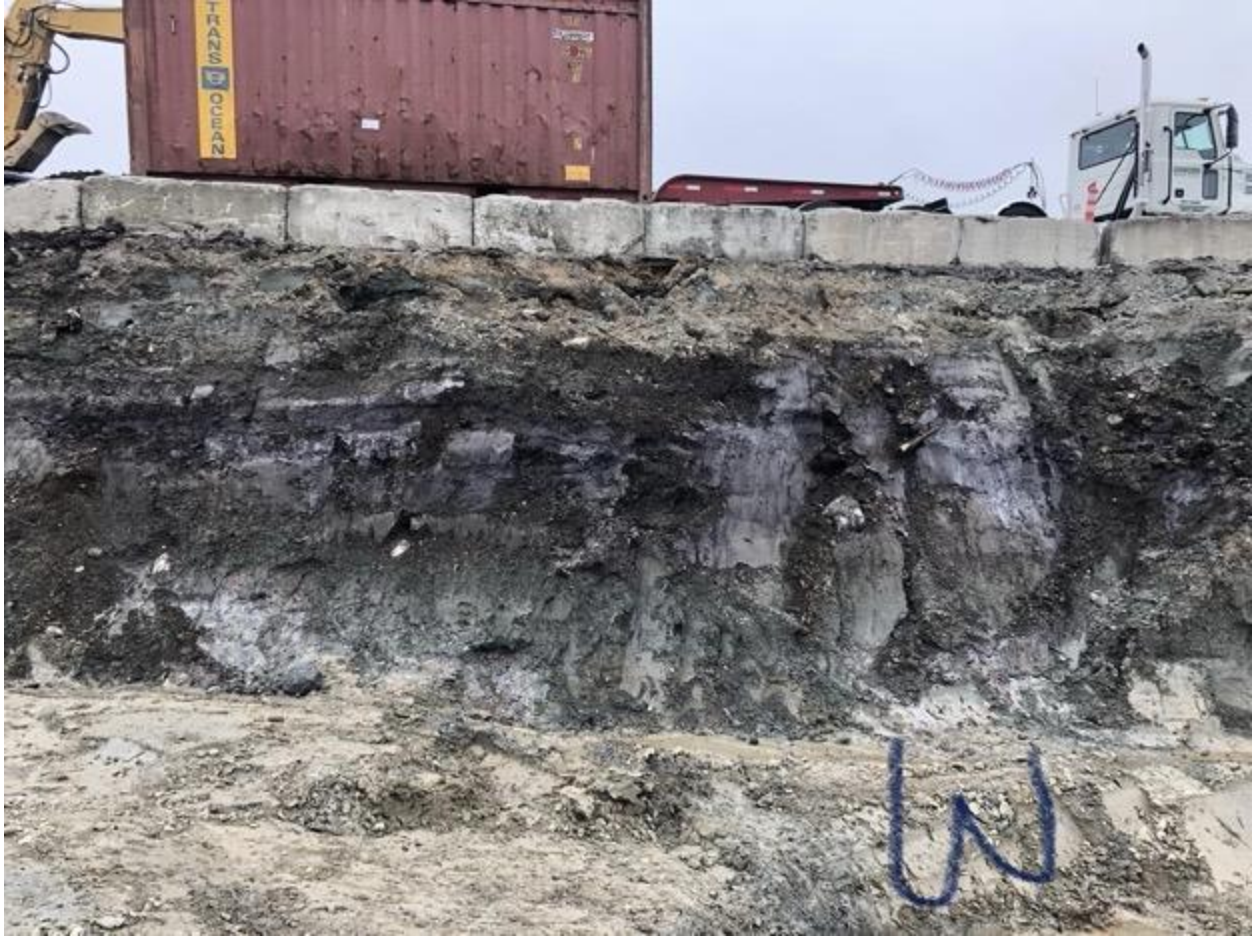
Figure 78. A photo of the approximate center of the site. This shows the eastern wall of the temporary road going down the site which the trucks use to park and have soil loaded. (photo taken facing West)
