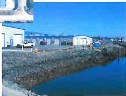
Figure 9. View of Web Lockers and Working Area
