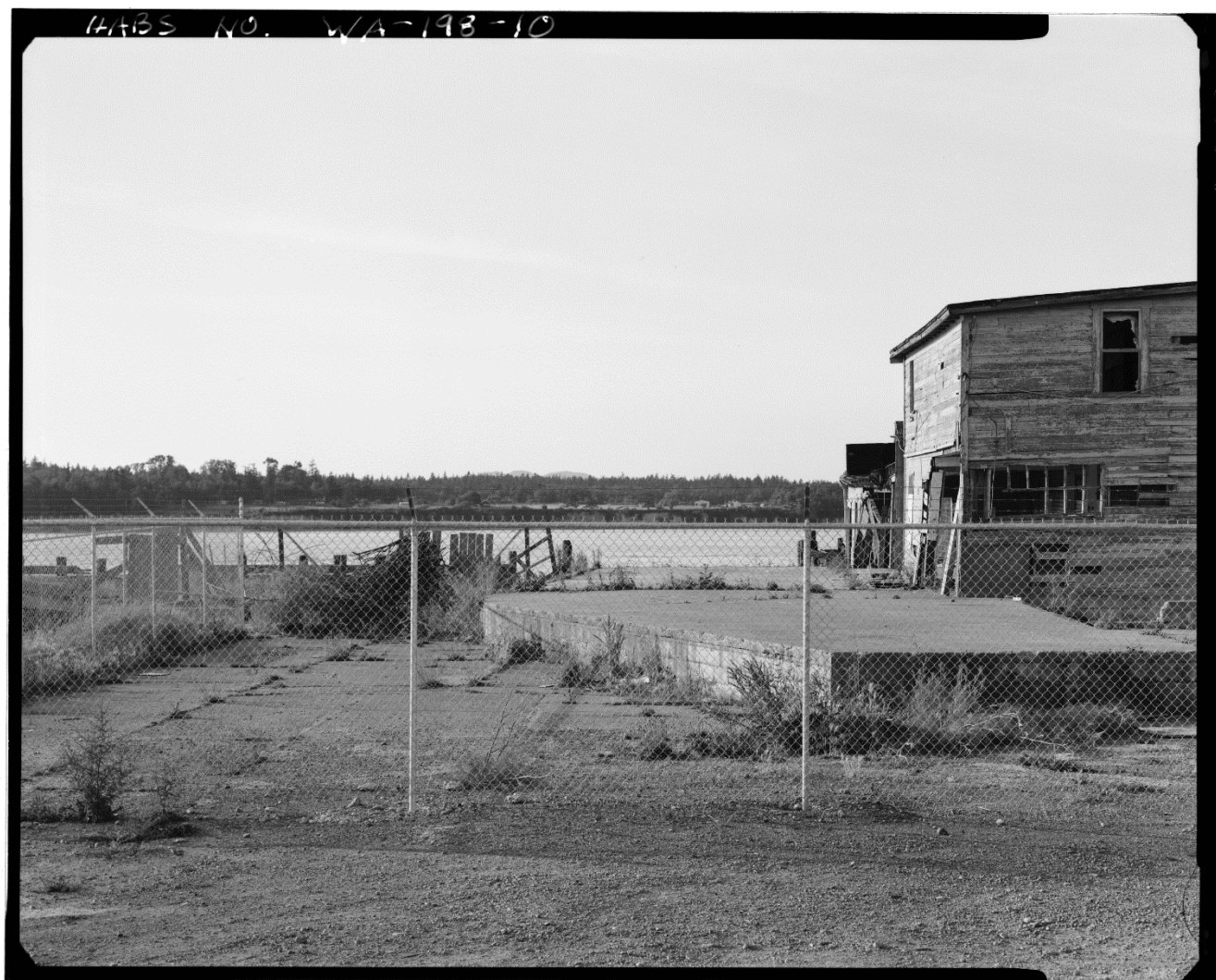
View east into the inner court between the Freight Warehouse and the Cold Storage Warehouse from the Sand and Gravel Wharf. Ferry slip is in the foreground. - Curtis Wharf, O & Second Streets, Anacortes, Skagit County, WA
