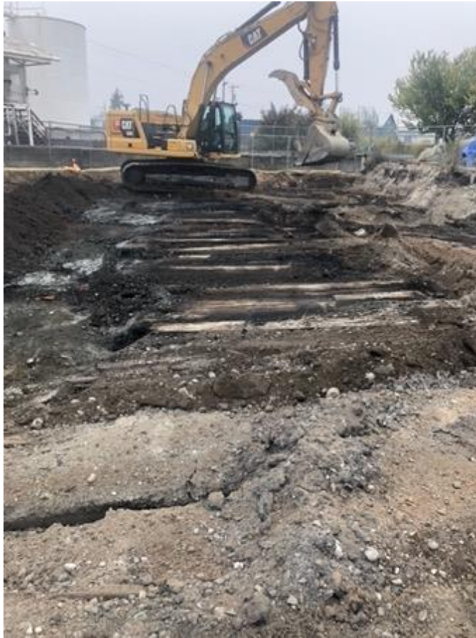
Figure 10. Coal Shed at Quiet Cove
