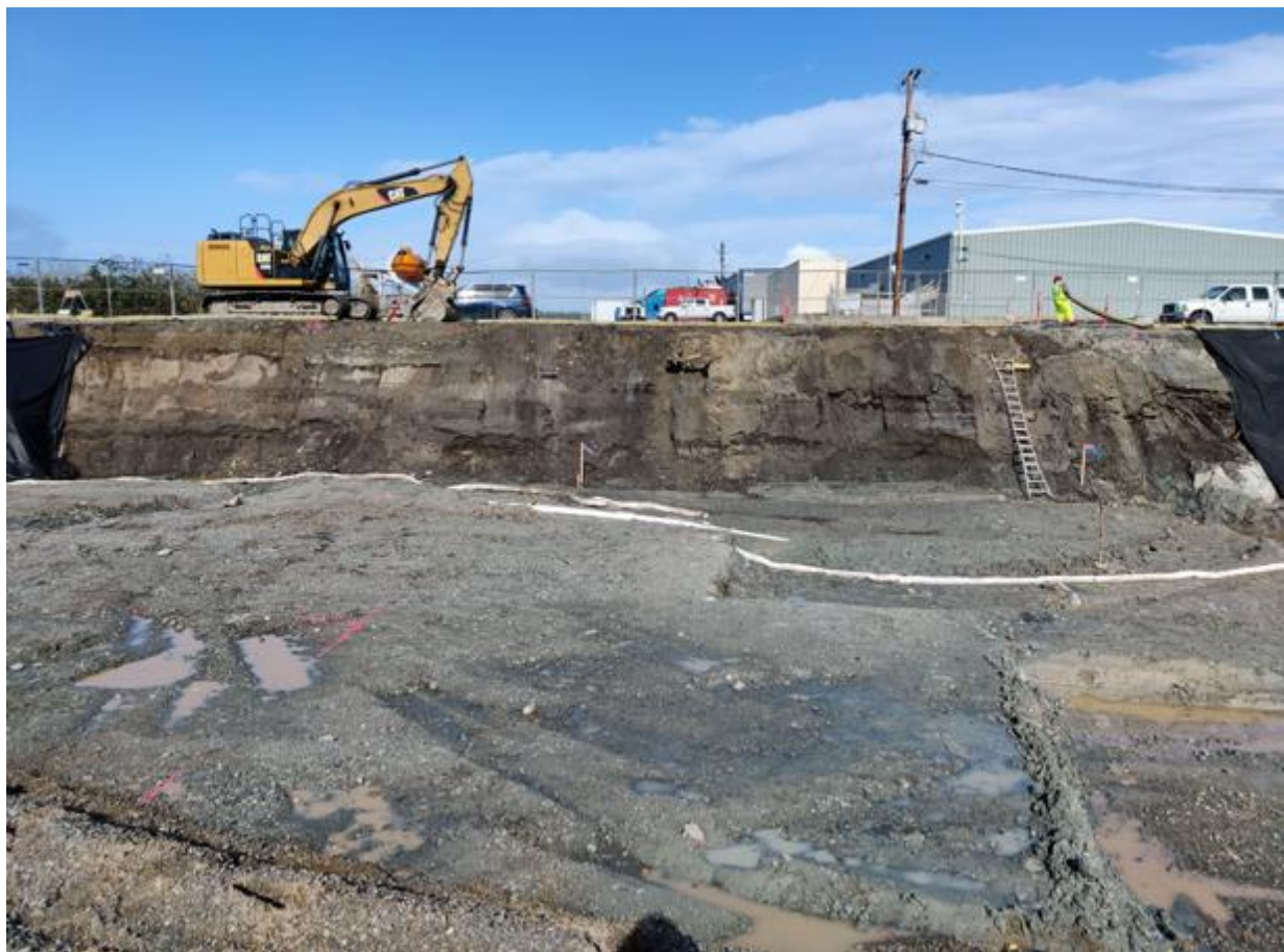
Figure 153. Excavation completion note contoured excavation margins.
