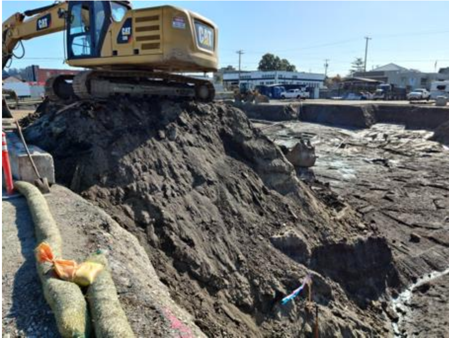
Figure 136. Overview of remaining soil to remove.
