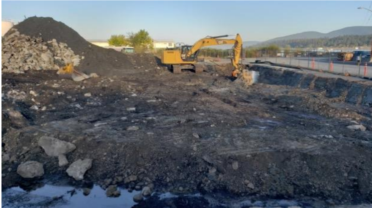
Figure 11. Site overview at start of day, facing WNW from eastern edge of site.
