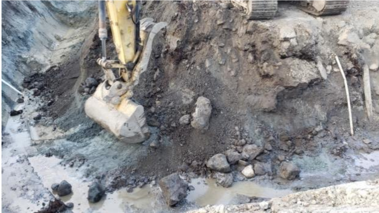
Figure 29. Boulder cluster in NE corner of excavations
