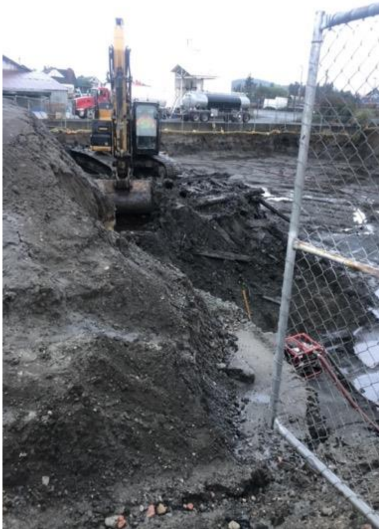
Figure 116. South facing photo of the western progress
