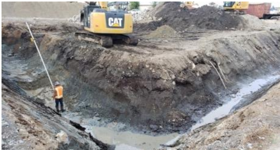
Figure 28. Start of day overview, facing SW from NE corner of project.
