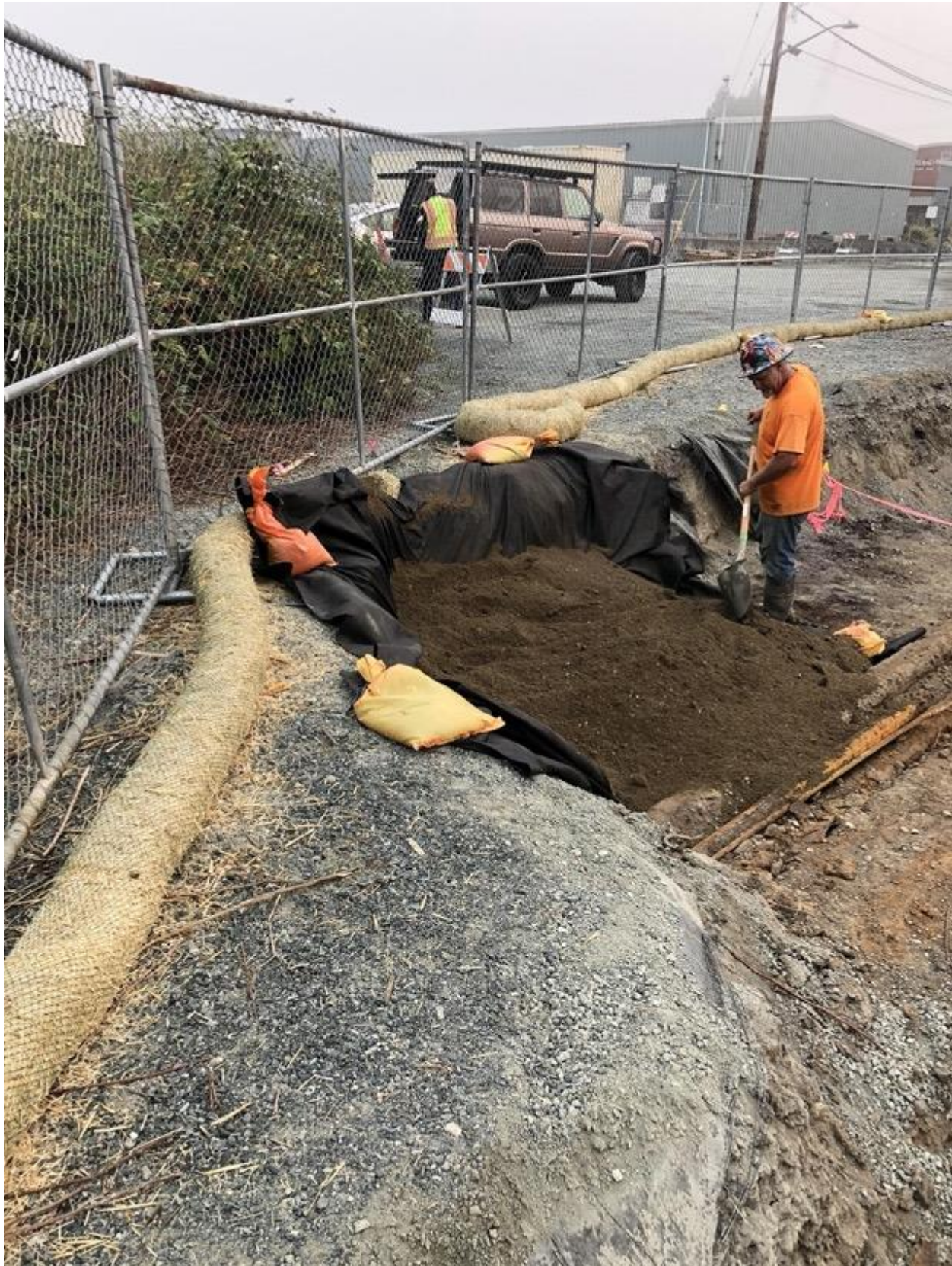
Figure 64. Backfilling conserved shell midden.
