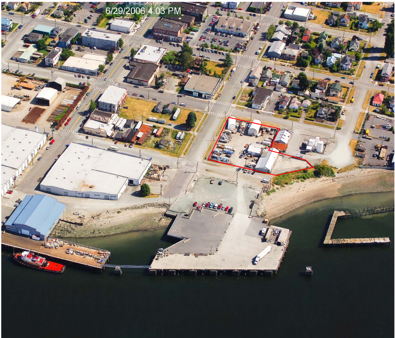
Overview of Quiet Cove and surrounding area - O & Second Streets, Anacortes, Skagit County, WA
