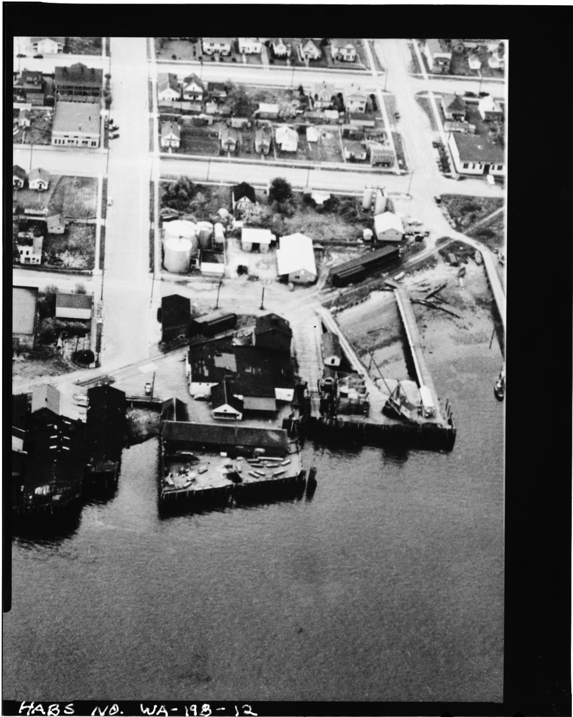
Photocopy of photograph (Original print, Port of Anacortes.) Brady's Anacortes Studio, Photographer, date unknown. Overview of Curtis Wharf and surrounding area. North section of main dock is intact; Sand and Gravel Wharf on the right. - Curtis Wharf, O & Second Streets, Anacortes, Skagit County, WA
