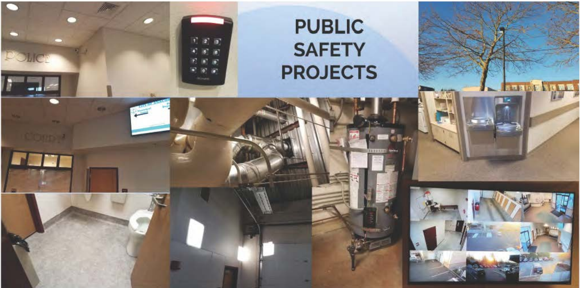
Water fountain upgrades, boiler venting replacement, camera upgrade and new installation (24 total units), court bathroom floor upgrade, exterior lighting, garage door openers replaced, hot water heater replacement, keypad and proximity (17 keypads), monitor installation, patrol monitor upgrade
