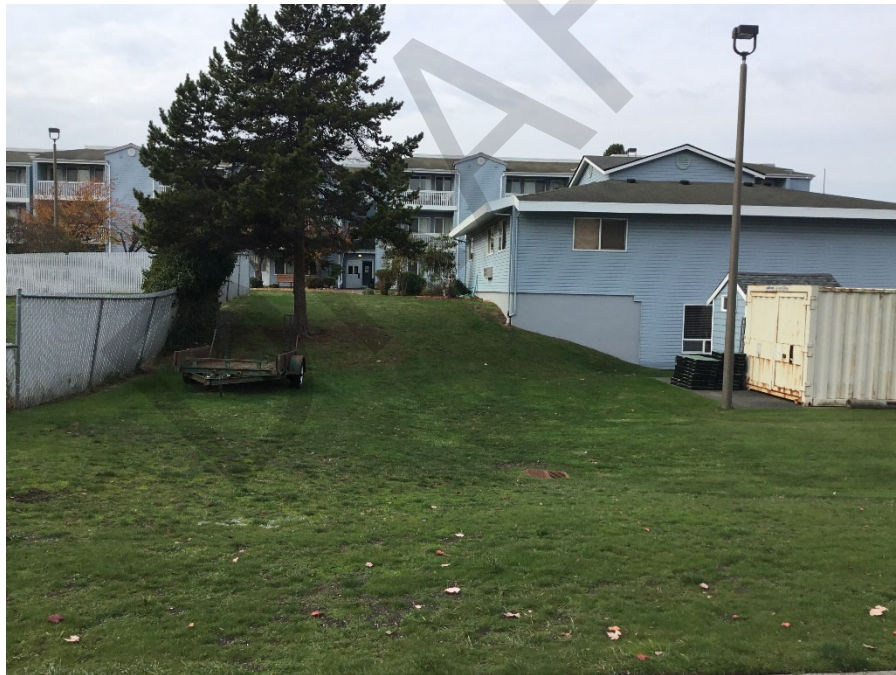
Photograph 14. An apartment building is located northeast of the dog park and within the northwestern corner of the proposed project area.
