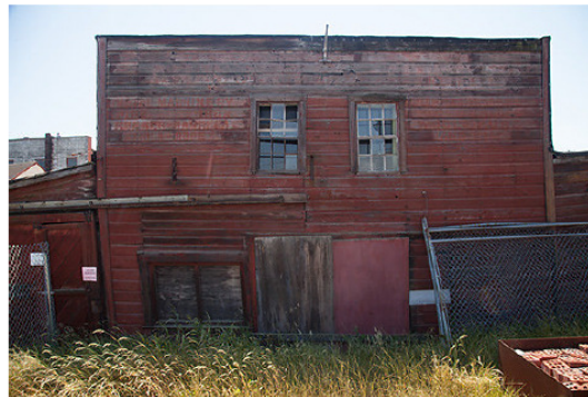
Figure 6. This photograph shows the north elevation wooden false front of the Livery Stable (19 June 2018).
