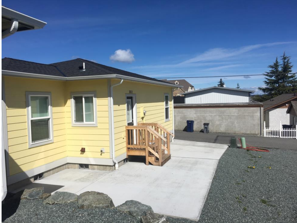
This is the subject property [Lot #4] that only has one off-street parking space
