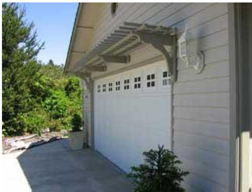
A decorative trellis over the garage door.
