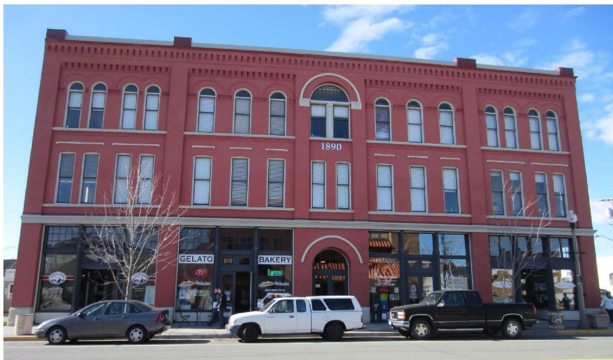
Figure 8 - The historic Wilson Hotel building
