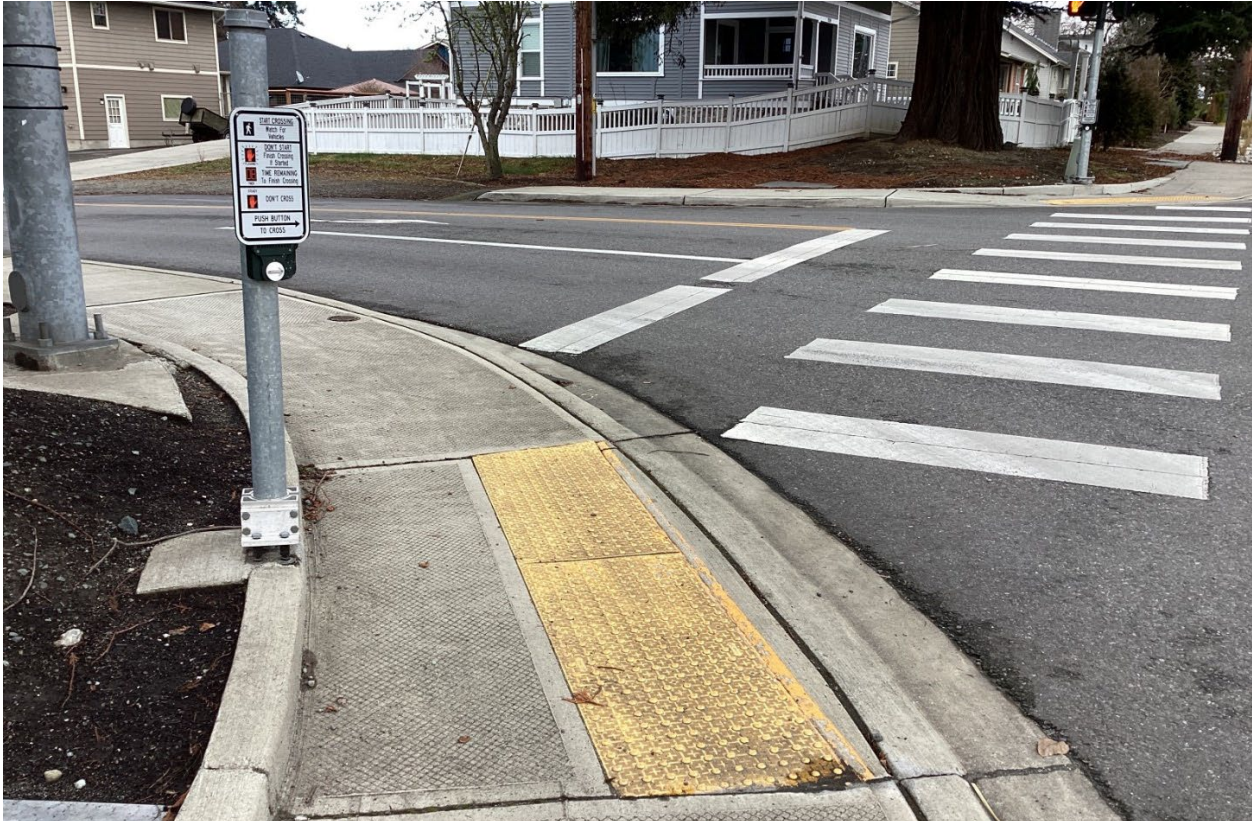
ADA-compliant accessible pedestrian signal in the city of Anacortes. Photo courtesy of Transportation Solutions, 2024.
