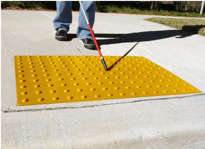
Compliant Truncated Domes
