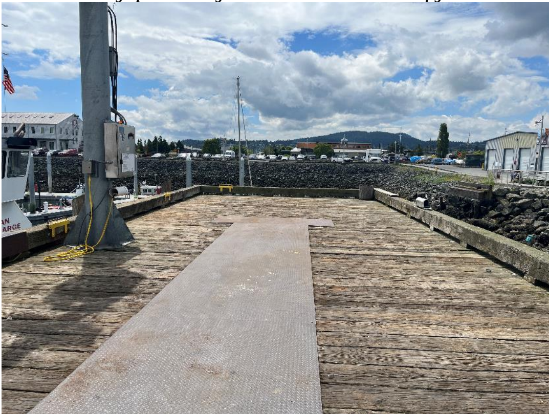
Photograph 8. Existing solid, creosote decking on T-Dock; crane to be salvaged and reinstalled.
