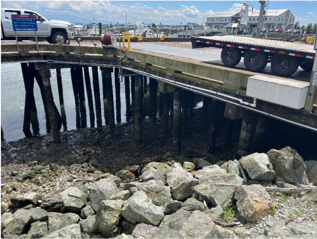
Photograph 7. Existing access to the T Dock to be reconfigured.
