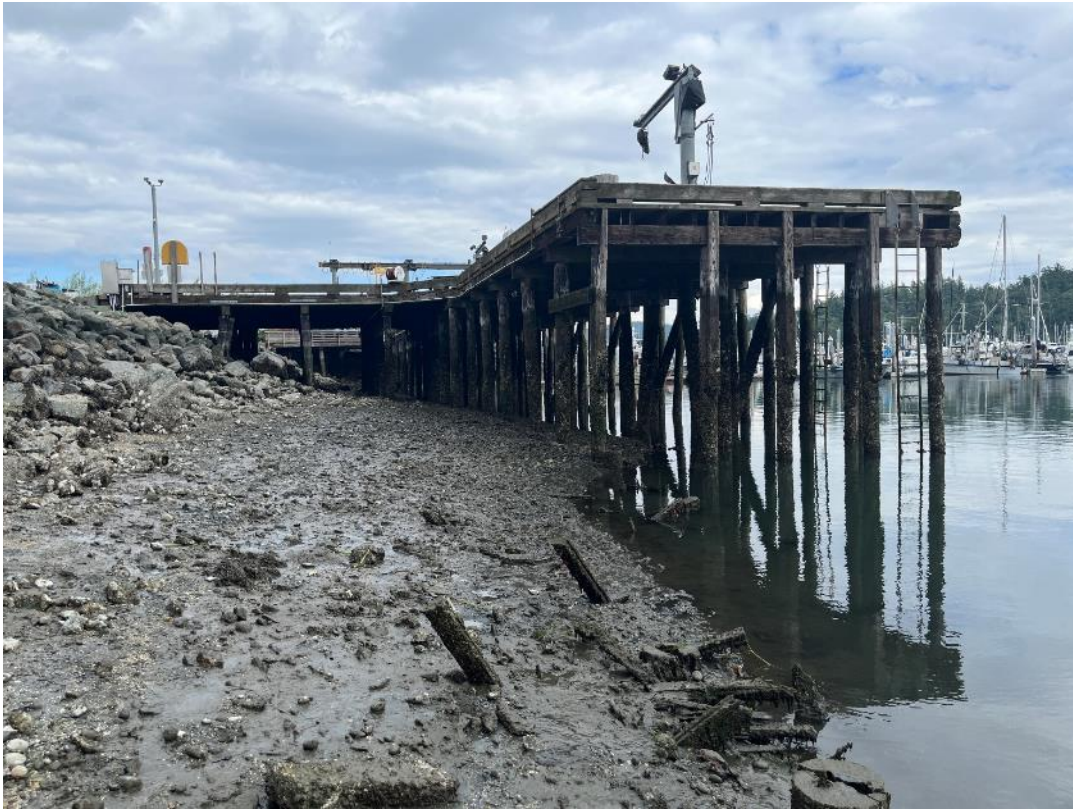
Photograph 3. Existing southern portion of the T Dock to be reconfigured; crane to be salvaged and reinstalled.
