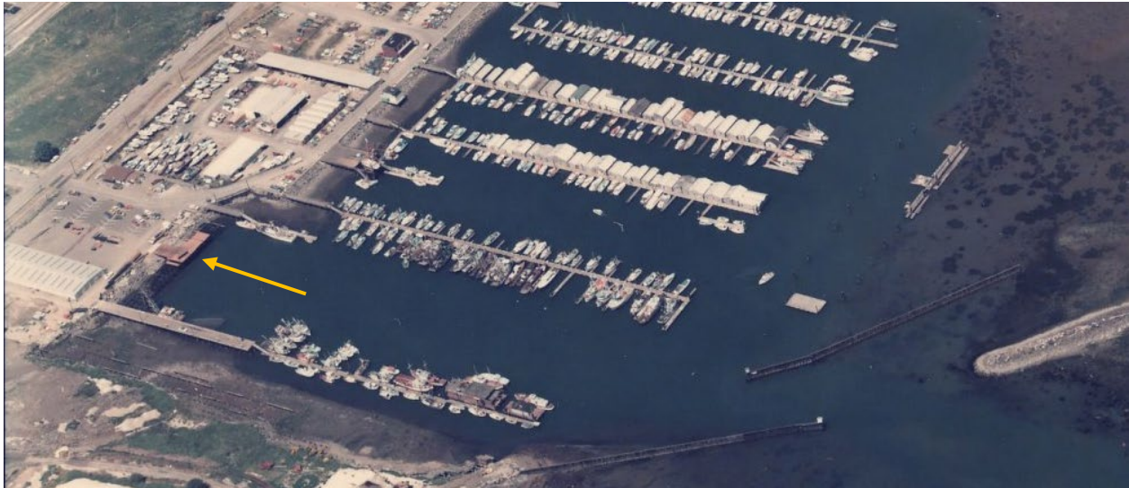
Photo circa 1977. “T-Dock” under construction.
