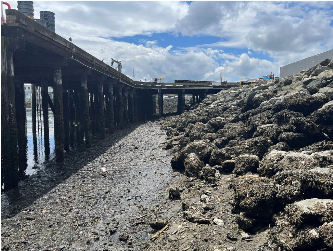
Photograph 15. Existing riprap shoreline within the northern portion of the T Dock that will be covered following reconfiguration.
