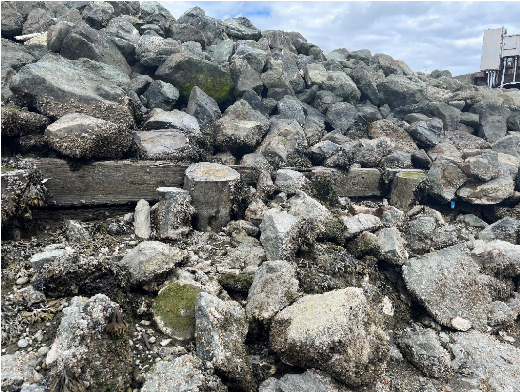
Photograph 17. Existing riprap shoreline within the southern portion of the T Dock that will be covered following reconfiguration; old timber bulkhead to remain.
