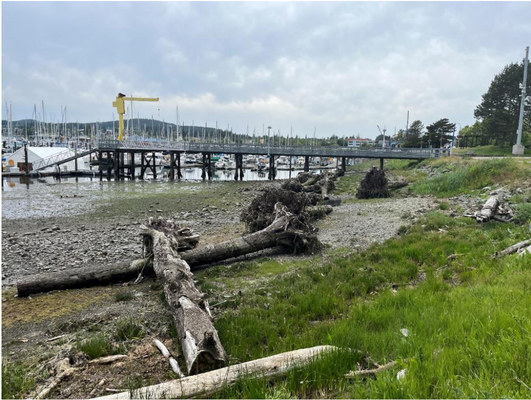
Photograph 19. Example large wordy debris installed as part of the mitigation for the A Dock replacement (2022) adjacent to the proposed mitigation location.
