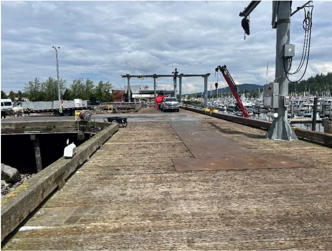
Photograph 9. Existing solid, creosote decking on T-Dock; cranes to be salvaged and reinstalled.
