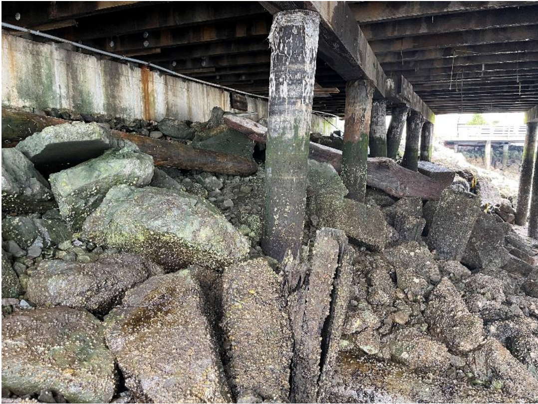
Photograph 11. Existing riprap shoreline located under the access to T Dock. existing pile and concrete retaining wall to be removed.
