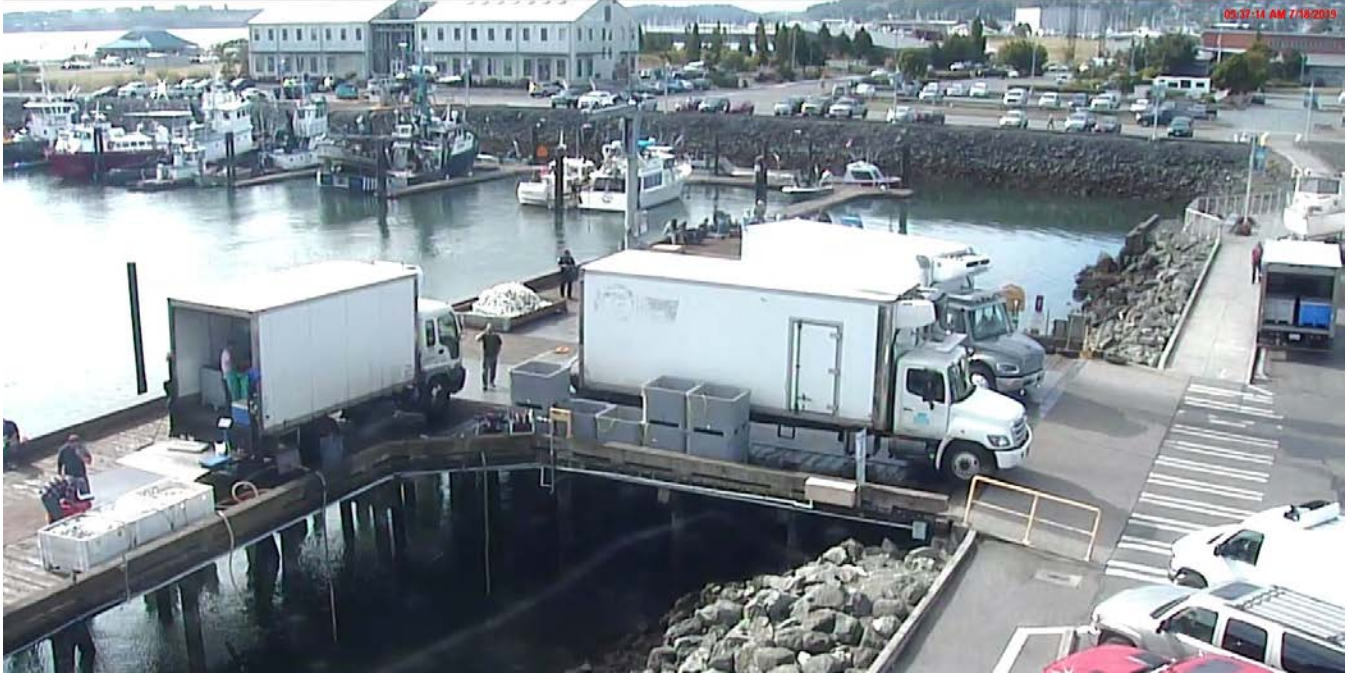
Photograph 2. Existing level of use on the existing T Dock.
