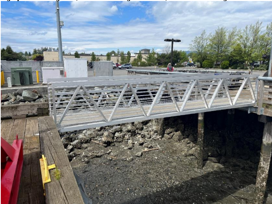
Photograph 10. Existing gangway at the norther end of the T Dock to be salvaged and reinstalled.
