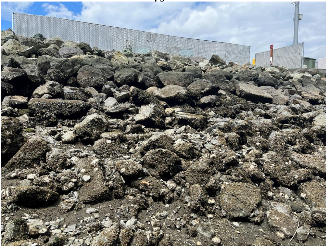
Photograph 16. Existing riprap shoreline within the northern portion of the T Dock that will be covered following reconfiguration.
