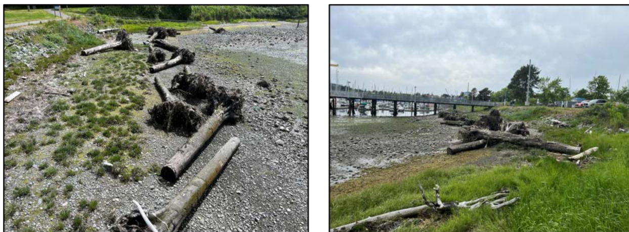
Figure 2. A Dock LWD placed in 2017 (photo June 2022).
