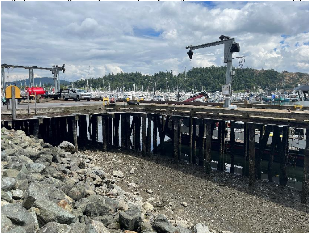
Photograph 6. Existing southern portion of the T Dock to be reconfigured; cranes to be salvaged and reinstalled.
