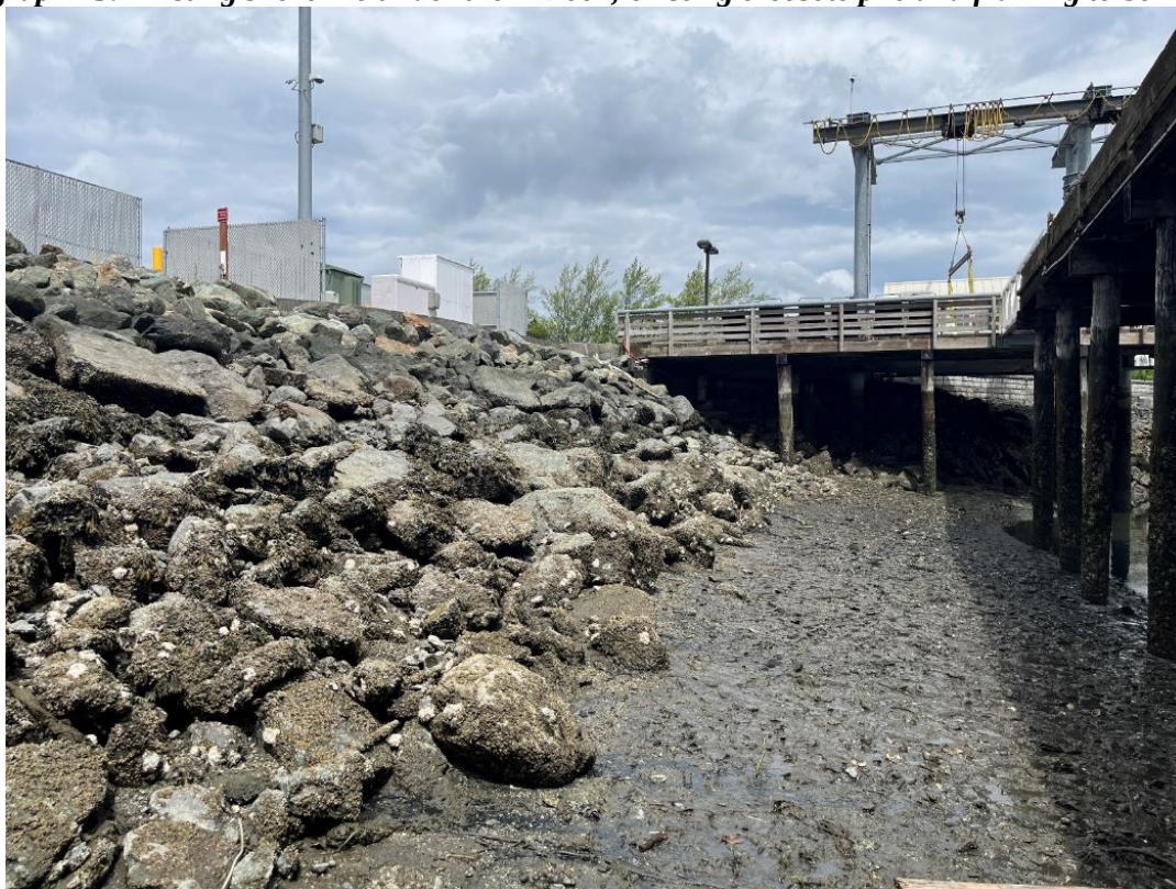
Photograph 14. Existing riprap shoreline within the southern portion of the T Dock that will be covered following reconfiguration.
