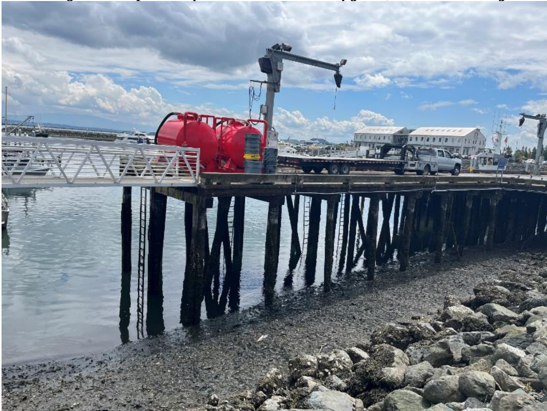
Photograph 4. Existing northern portion of the T Dock to be reconfigured; cranes and gangway to be salvaged and reinstalled.
