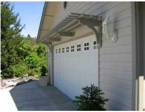
A decorative trellis over the garage door.
