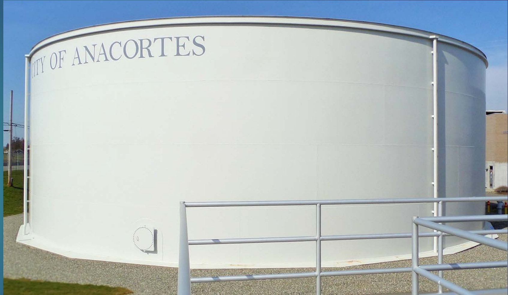
2.1-Million-Gallon Clearwell at Water Treatment Plant
