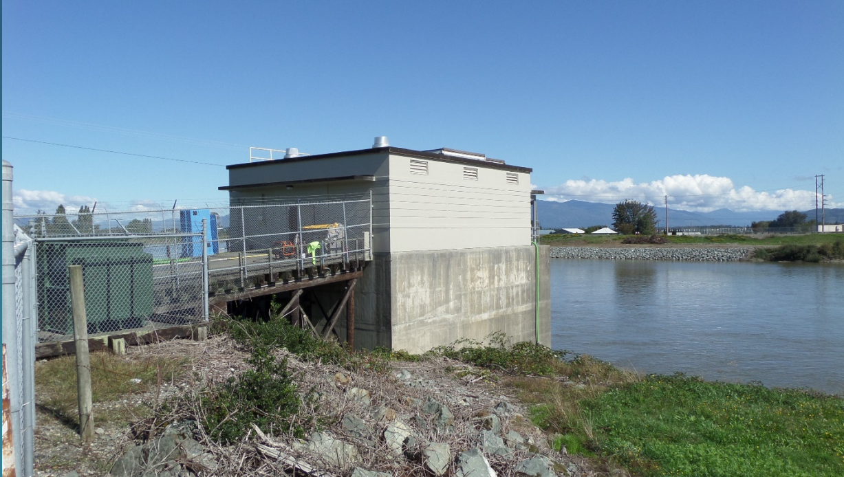
Intake Pump Station
