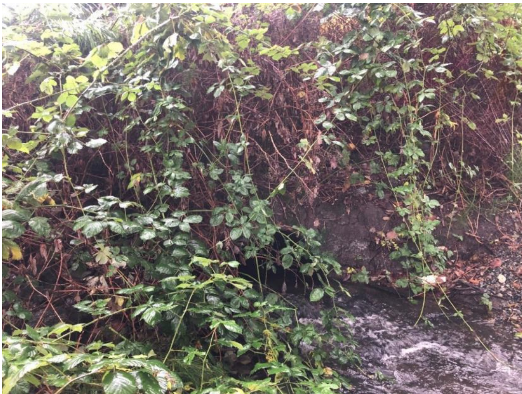
Ace of Hearts Creek culvert outlet on the north end of Ace of Hearts Rotary Park
