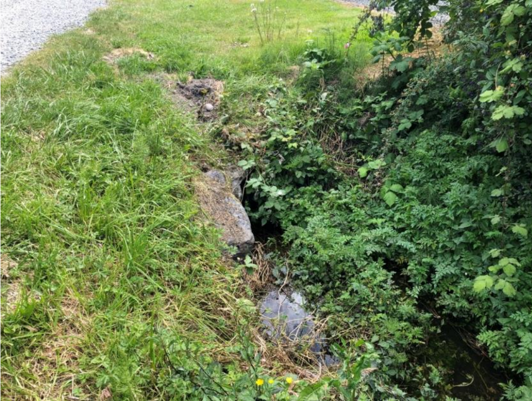
Ace of Hearts Creek culvert inlet, east side of entrance road to Ace of Hearts Rotary Park from H Avenue
