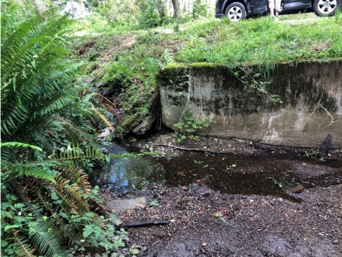
Cranberry Creek flows from left to right along Cranberry Creek Road prior to its inlet to the piped system
