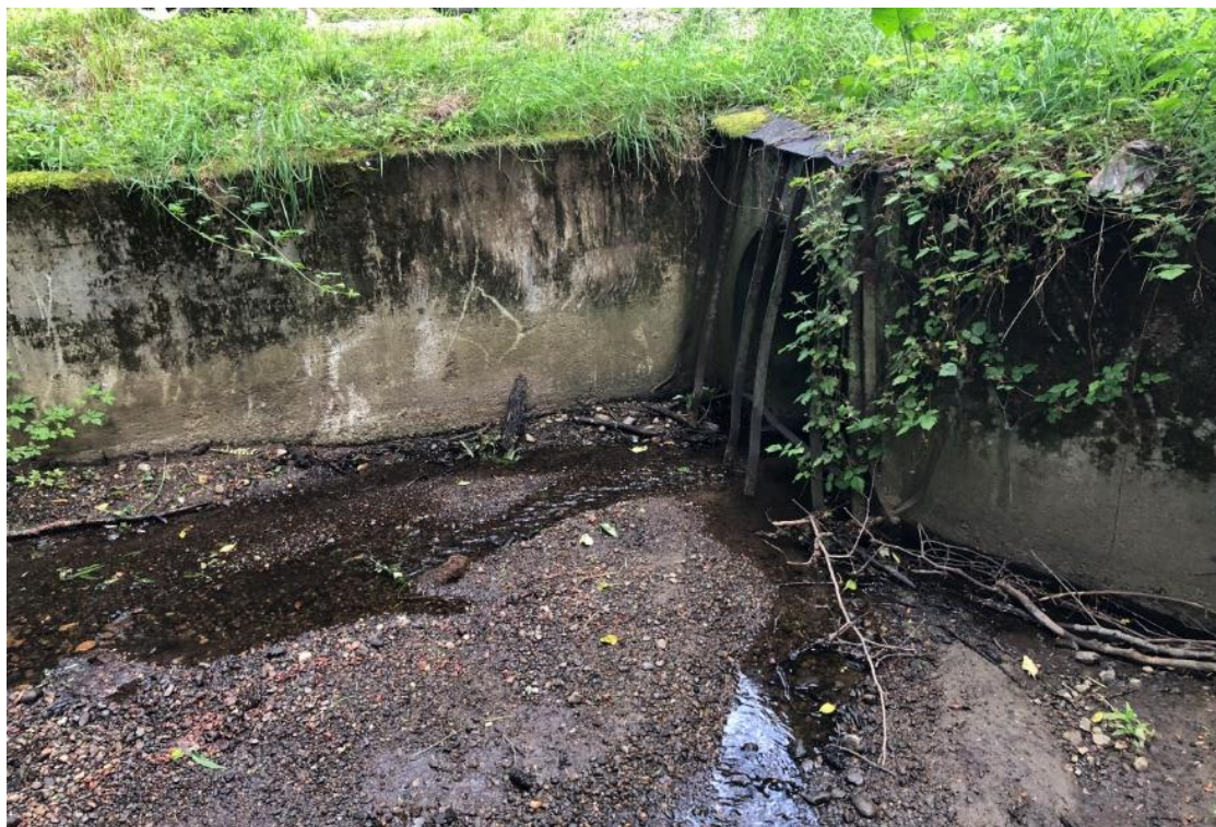
Cranberry Creek at culvert inlet to piped system at Cranberry Lake Road
