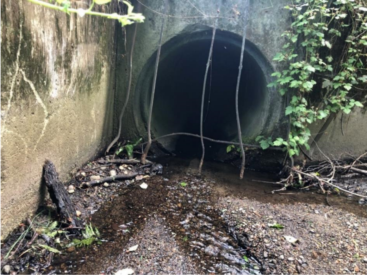
Inlet to the piped Cranberry Creek system at Cranberry Creek Road
