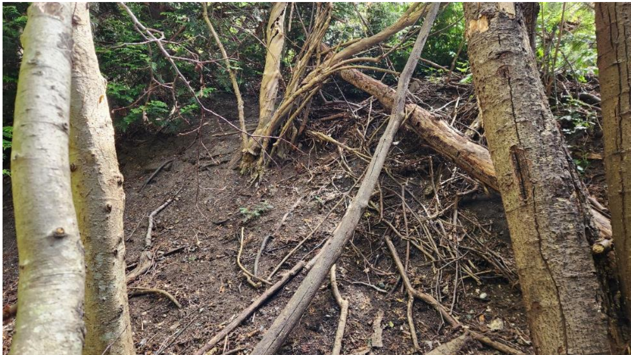
Erosion, exposed tree roots, falling trees, and high-water line upstream of culvert at Clyde Way
