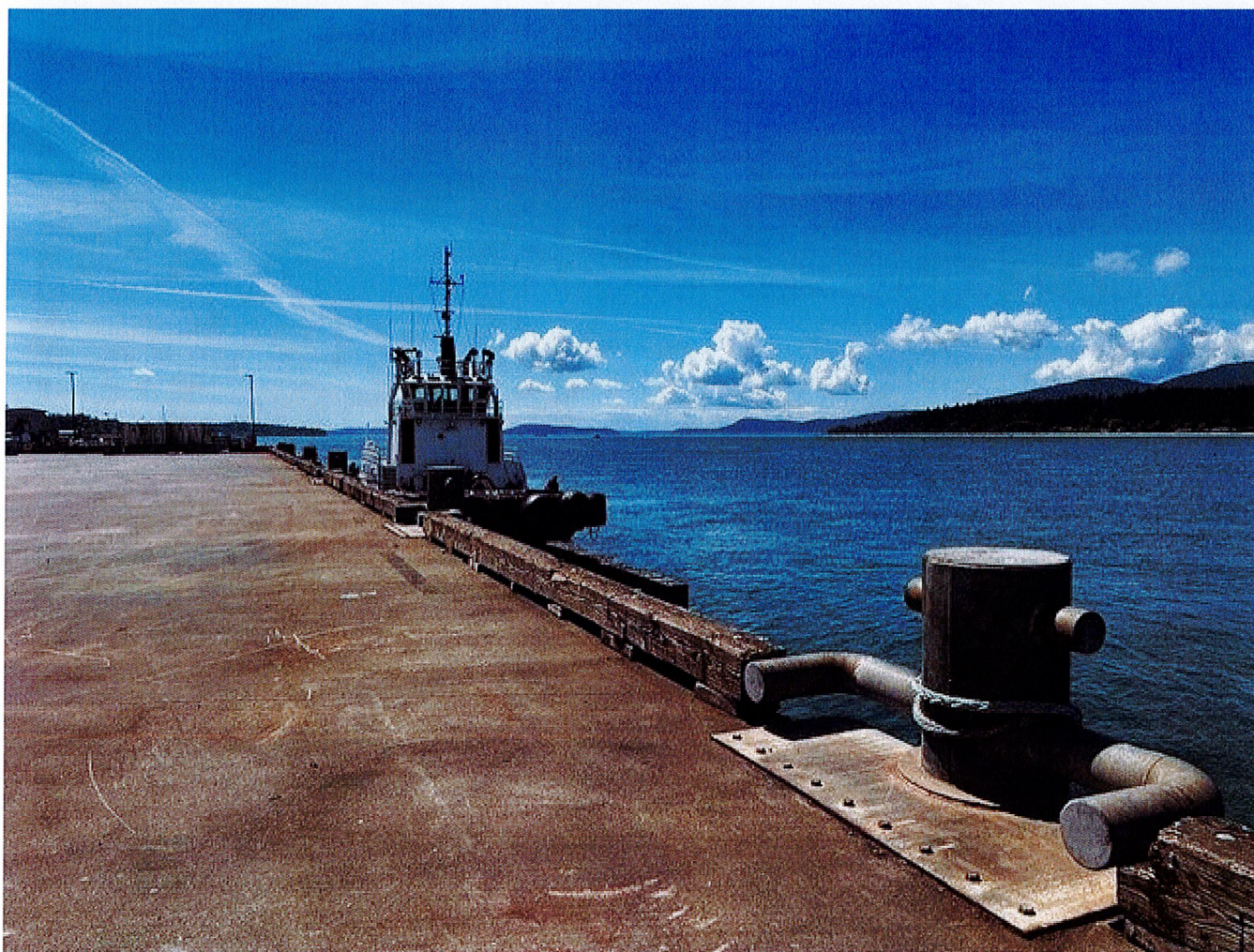
Figure 4: Curtis Wharf Looking West
