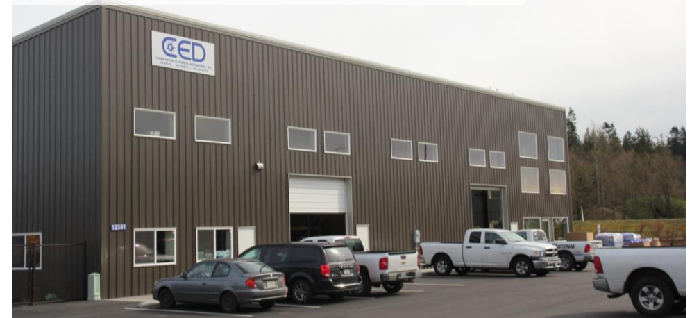
New Industrial Near Sharpe's Corner (2017)
