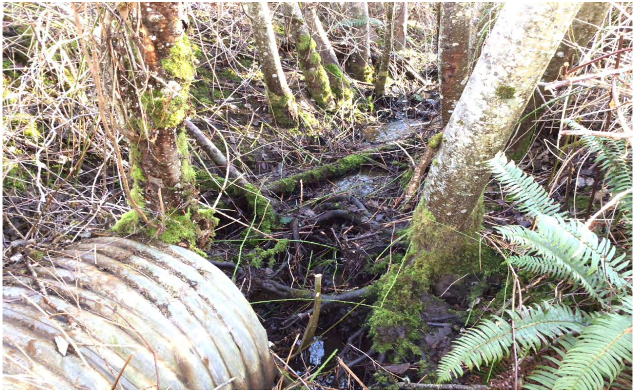
Photo 8. Howard Creek conditions at culvert junction on parcel 19971.
