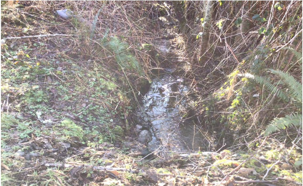
Photo 7. Howard Creek conditions at culvert junction on parcel 19972.
