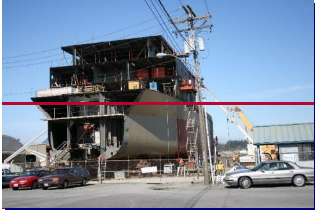
Ship Building at Marine Terminal
