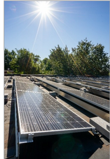
Solar panel installation.
