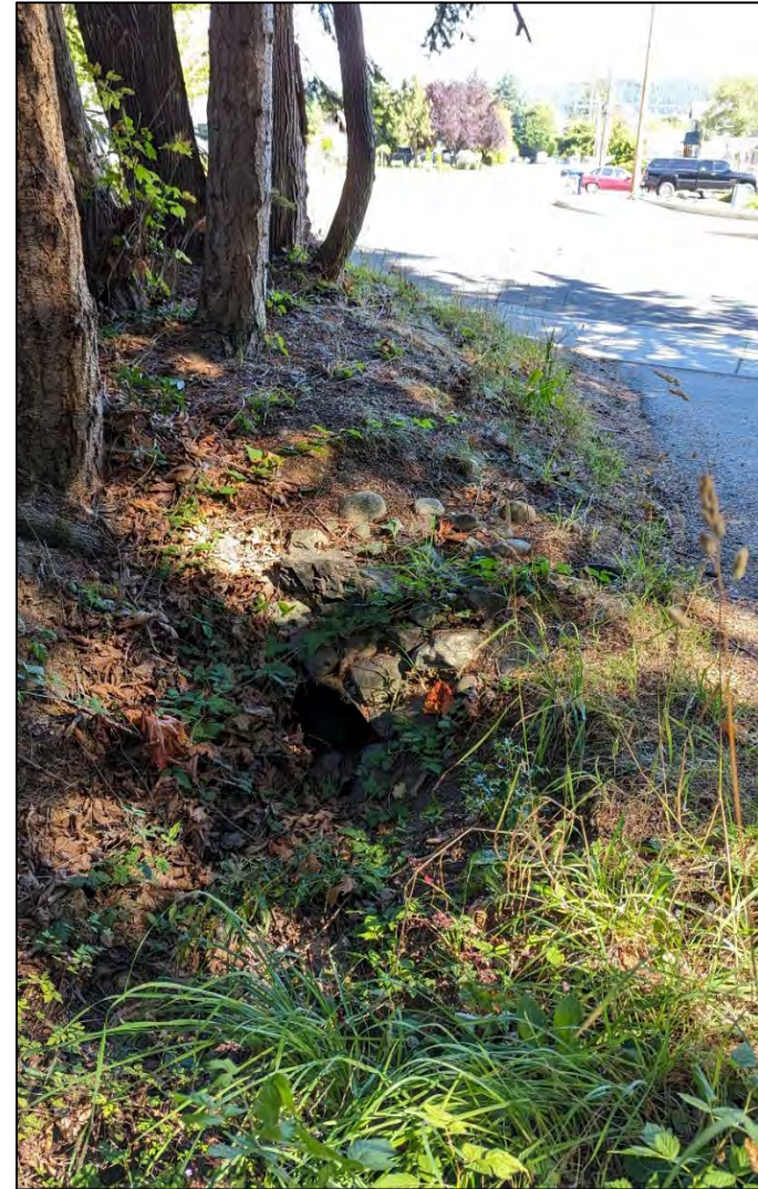
Photo 11. Culvert southeast of intersection of 17 th Street and Alaska Avenue, facing north.
