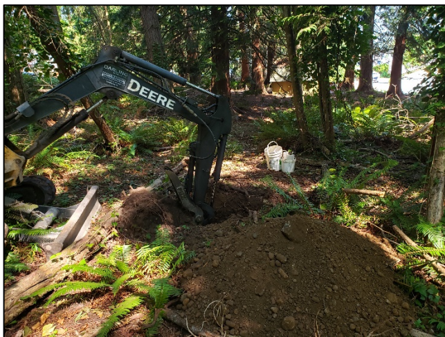
Above: Excavation of TP-4. Conditions as pictured are generally typical of site conditions.
