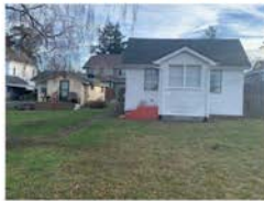
31st Street House- One Large Family
